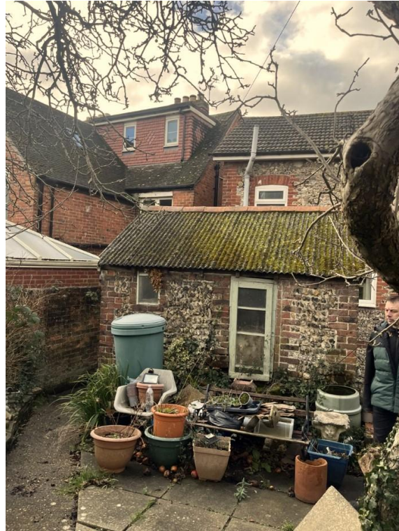
Rear of 14 Bridgefoot Path showing how Number 15 interacts with the proposal, Number 14. The original structure of the proposal is a mix of flint and brick. The asbestos roof and structure of the current outbuilding is in poor condition and structurally unsound.
