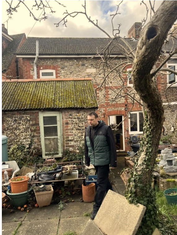
Rear of 14 Bridgefoot Path showing how Number 15 interacts with the proposal, Number 14. The original structure of the proposal is a mix of flint and brick. The asbestos roof and structure of the current outbuilding is in poor condition and structurally unsound.
