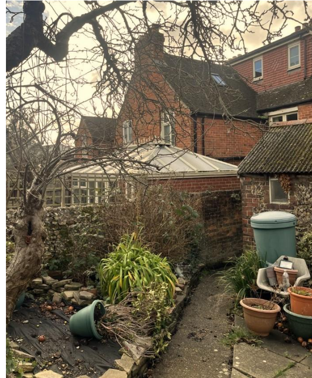
Rear of 14 Bridgefoot Path showing how Number 15 interacts with the proposal, Number 14. The original structure of the proposal is a mix of flint and brick. The asbestos roof and structure of the current outbuilding is in poor condition and structurally unsound.
