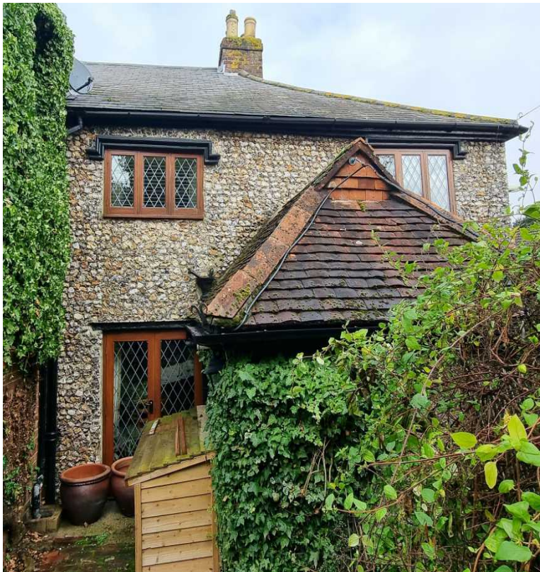
Left: A portion of the side elevation is also knapped flint.
