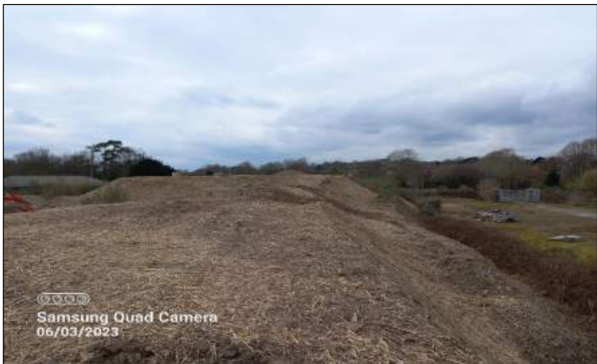
Photo 2: View looking west across the site.
