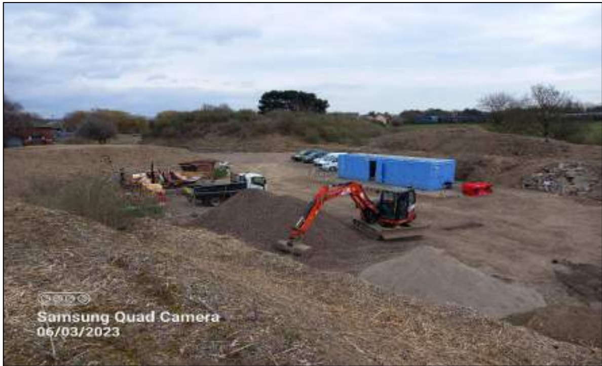
Photo 3: View looking east across the site.
