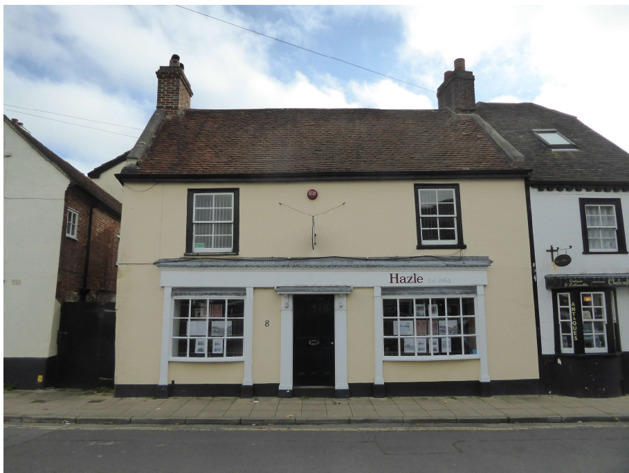
4. 8 South Street existing beige façade
