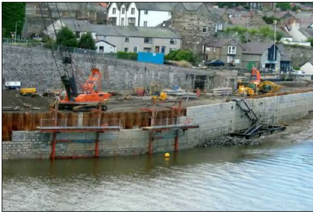
PRE-CAST CONCRETE PANELS TEXTURED WITH NATURAL STONE FINISH (PHOTO FROM RPC CONTRACTS LTD)
