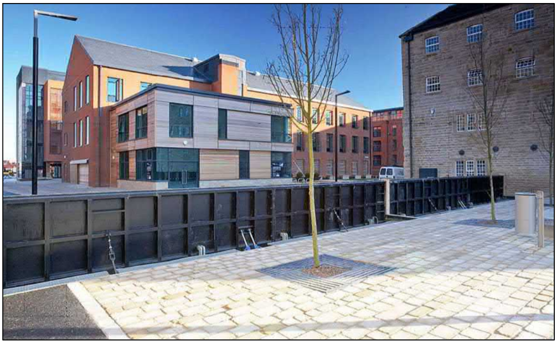
DEPLOYED FLIP-UP FLOOD BARRIER (PHOTO FROM FLOOD CONTROL INTERNATIONAL LTD)
