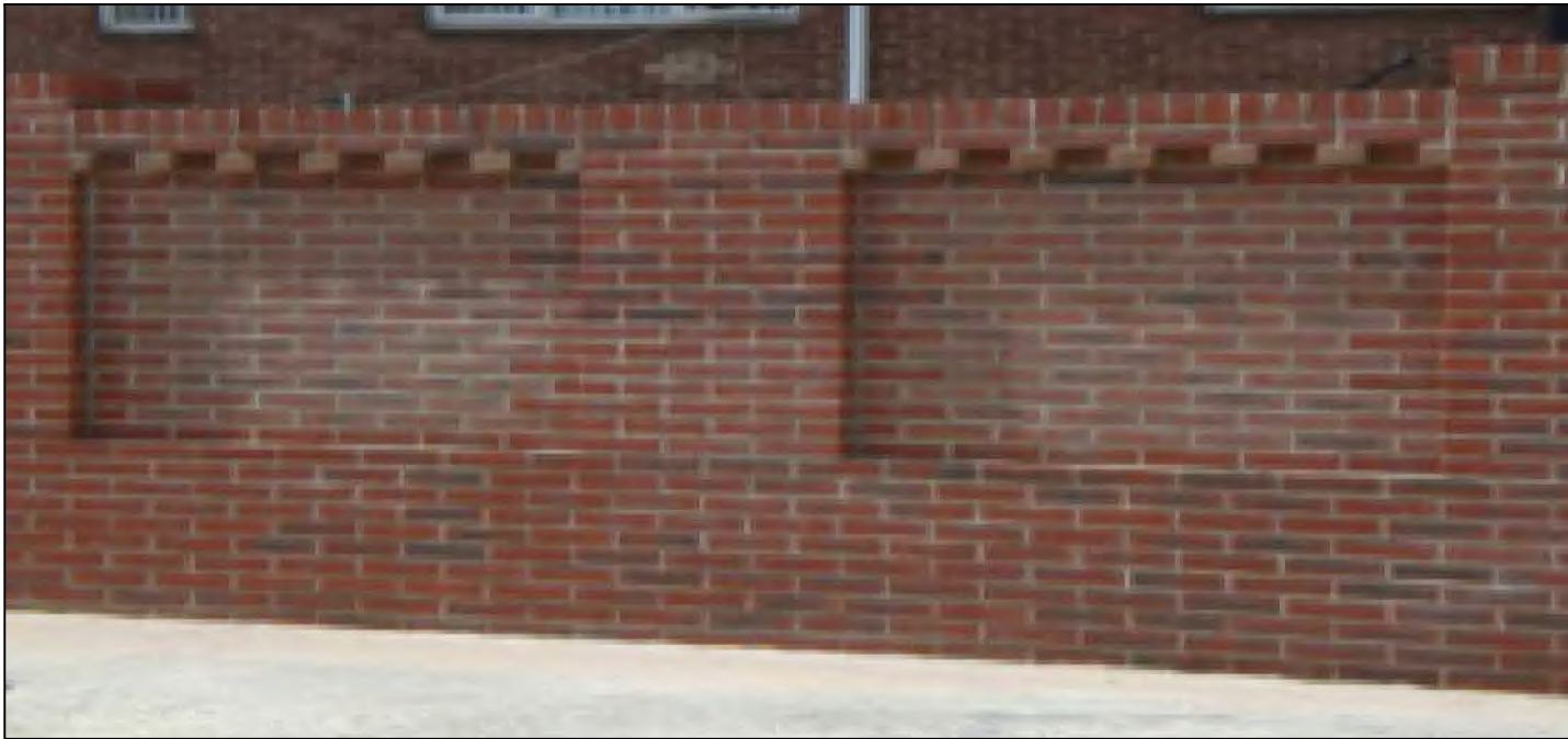
RECESSED BRICK CLADDING
