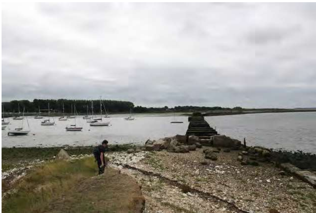
Photo 5: Remains of the railway bridge to Havant
