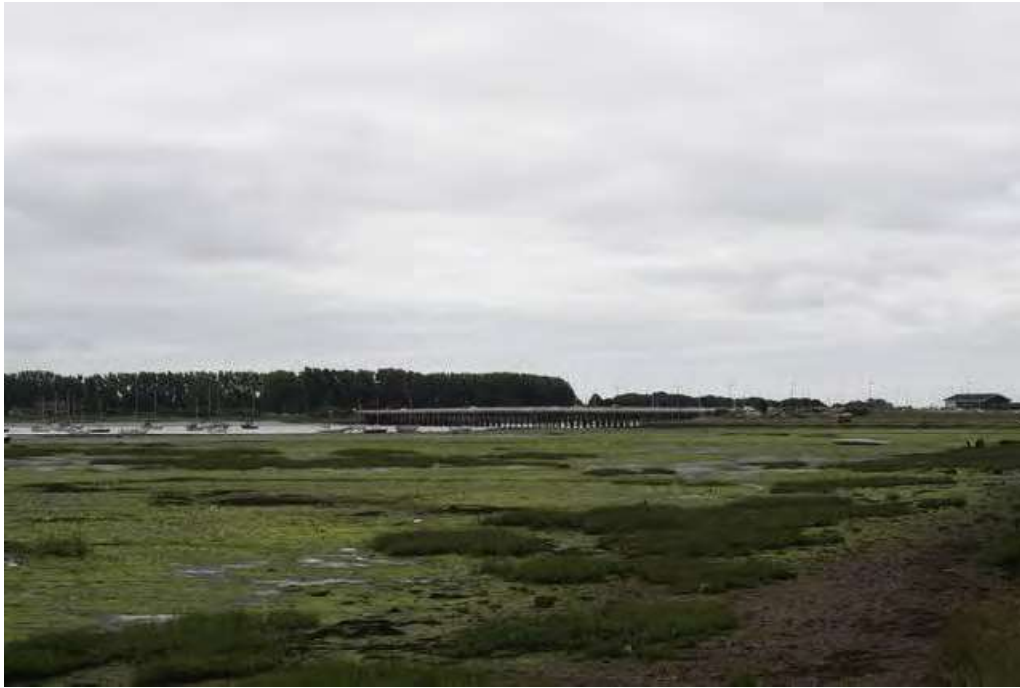
Photo 19: View towards Langstone Bridge
