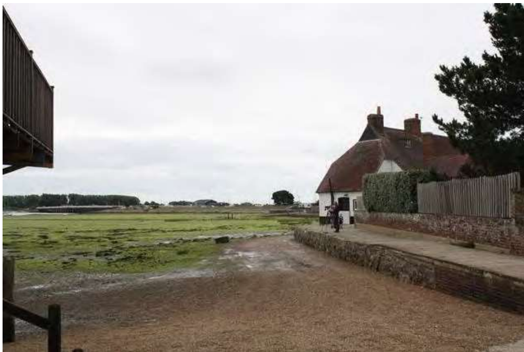
Photo 15: Panoramic view, west of the Old Mill
