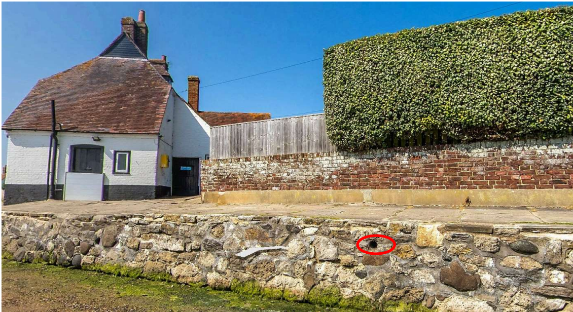
Figure 3-6: Example of an existing drainage conduit from behind a boundary wall (Frontage 5)
