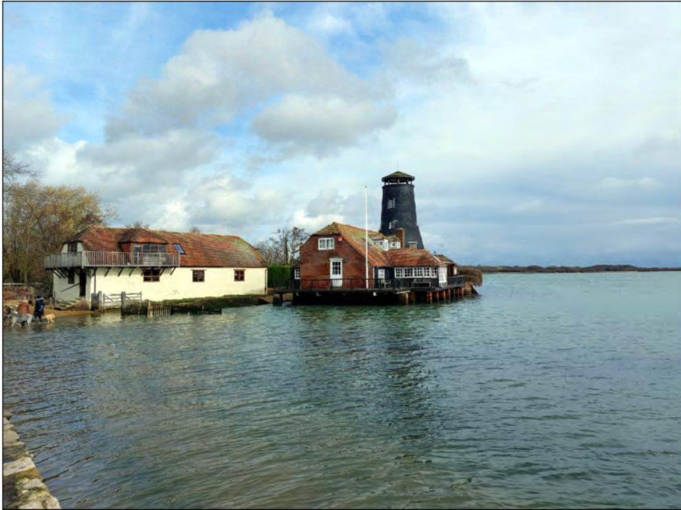
Photo 11) View looking north-east past The Old Mill (NHLE 1340200) from the south-east harbour front
