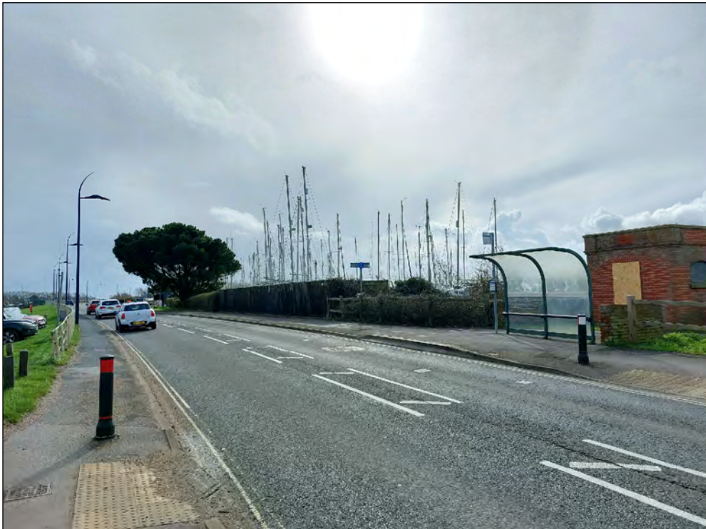
Photo 5) View looking south-west across Langstone Sailing Club and the point where Frontage 2 meets Langstone Road
