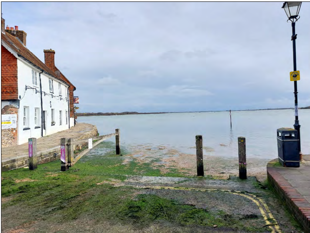
Photo 10) View looking south-east across the Langstone High Street slipway
