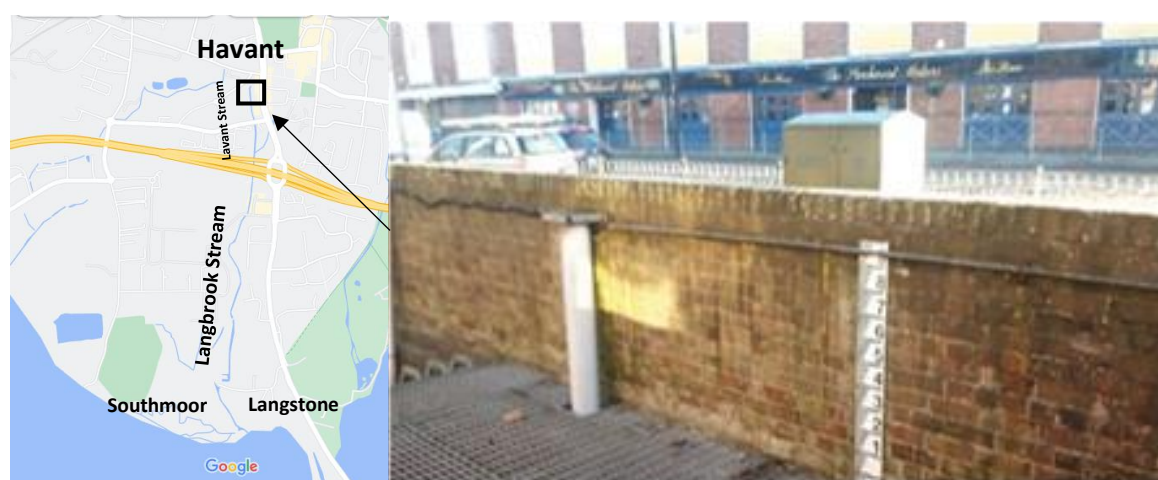
Figure 3: Havant levels gauge (Site of decommissioned flow gauge)
