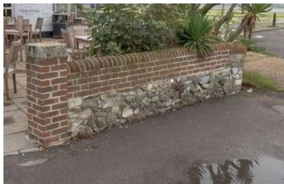
Figure 3-3: Existing wall proposed to be left in place at northern end of sub-unit 3b (photo ©2019 Google Maps)
