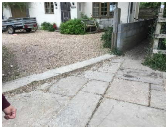
Figure 3-16: Sub-unit 3f flood gate location across property vehicle access
