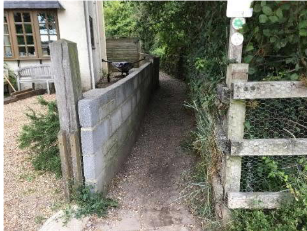
Figure 3-14: Sub-unit 3l existing wall
