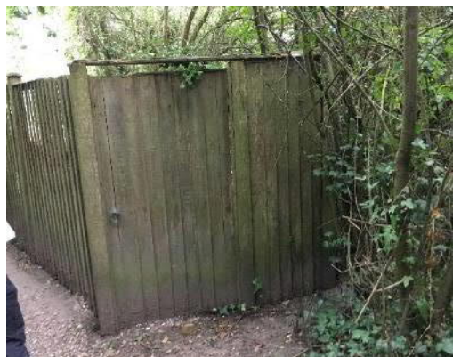
Flood gate no. 9 location
