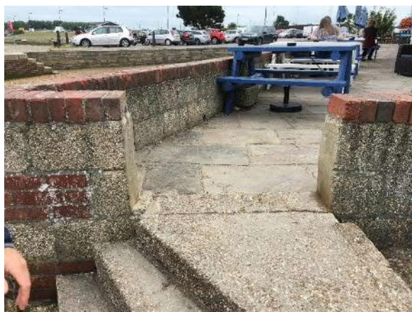
Figure 3-4: Sub-unit 3d to 3e existing wall in front of Ship Inn
