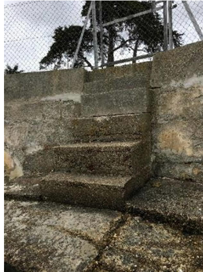
Figure 4-7: Sub-unit 1b access steps
