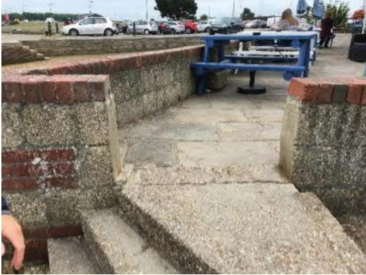
Flood gate no. 1 location
