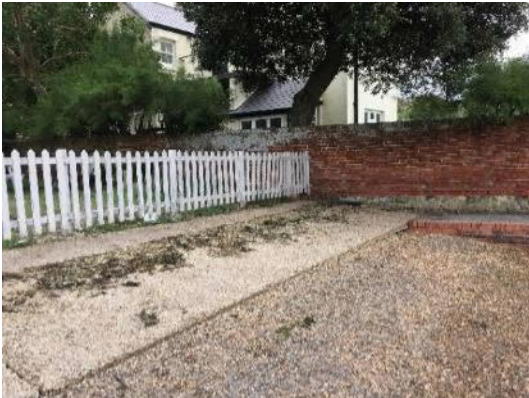
Flood gate no. 2 location – along fence line
