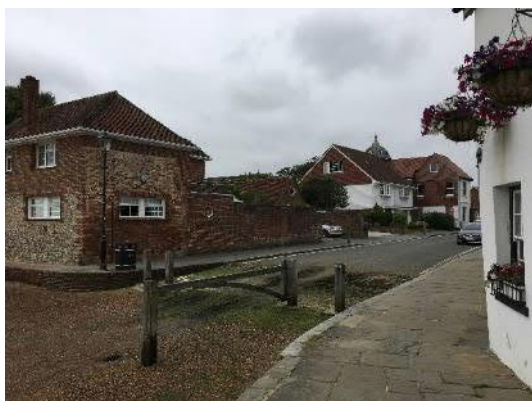
Flood gate no. 6 location
