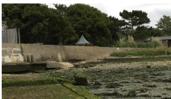
Figure 4-6: Eastern end of sub-unit 1b seawall
