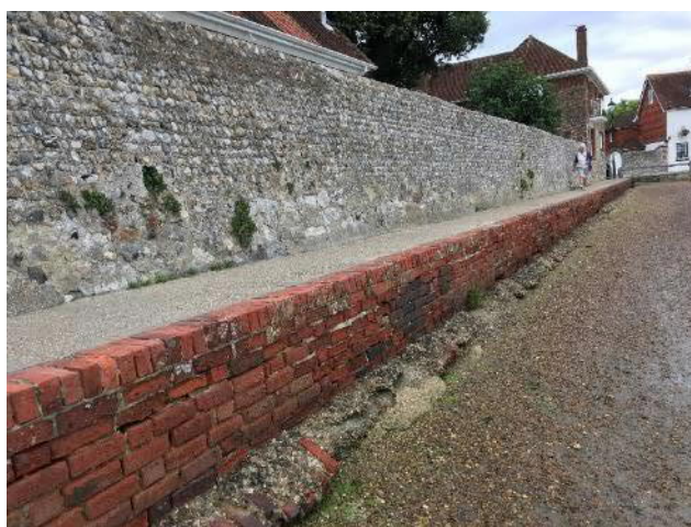
Figure 3-6: Sub unit 3f to 3h showing existing seawall apron
