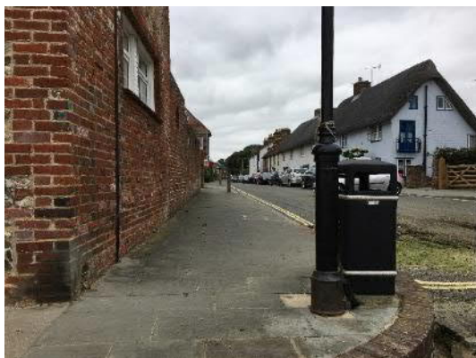
Flood gate no. 5 location
