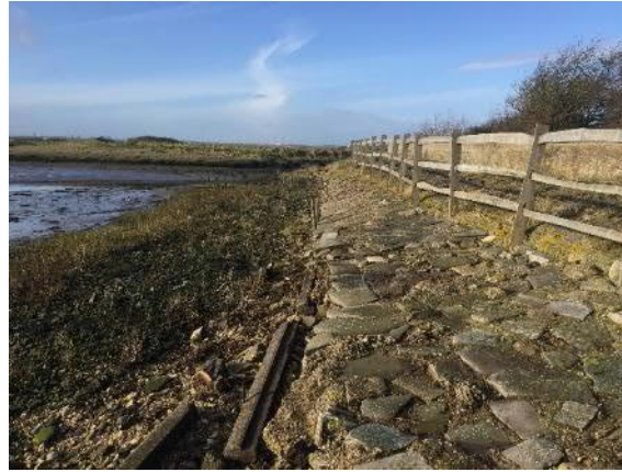
Figure 4-2: Structure 1 sub-unit ODU1b West
