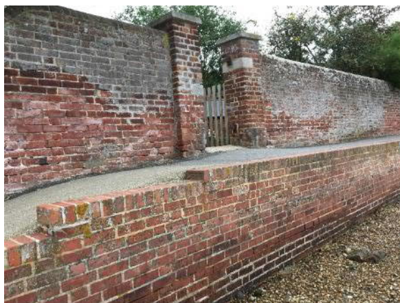
Figure 3-9: Sub unit 3f to 3h flood gate location
