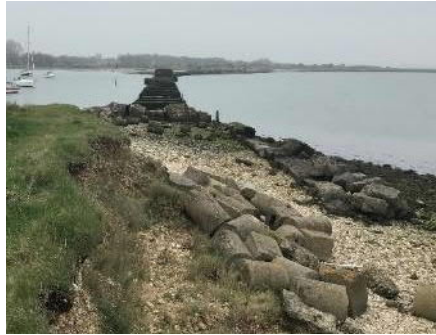
Figure 4-9: Concrete rubble located on the spit
