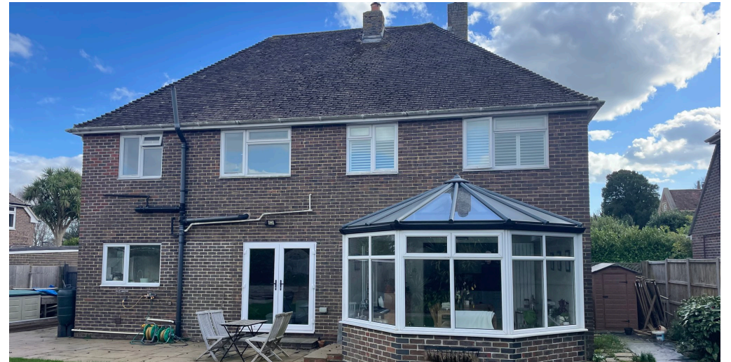
The existing rear elevation of Rosemead
