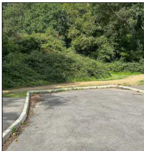
Photograph 2: End of Road at Merritt Way
