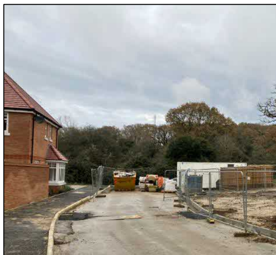
Photograph 3: End of Road at Wilkes Way
