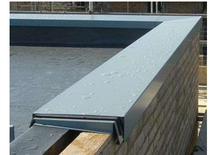
4 Flashings: Dark grey metal cladding
