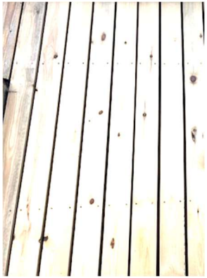
1 Walls: Vertically Laid Timber Cladding
