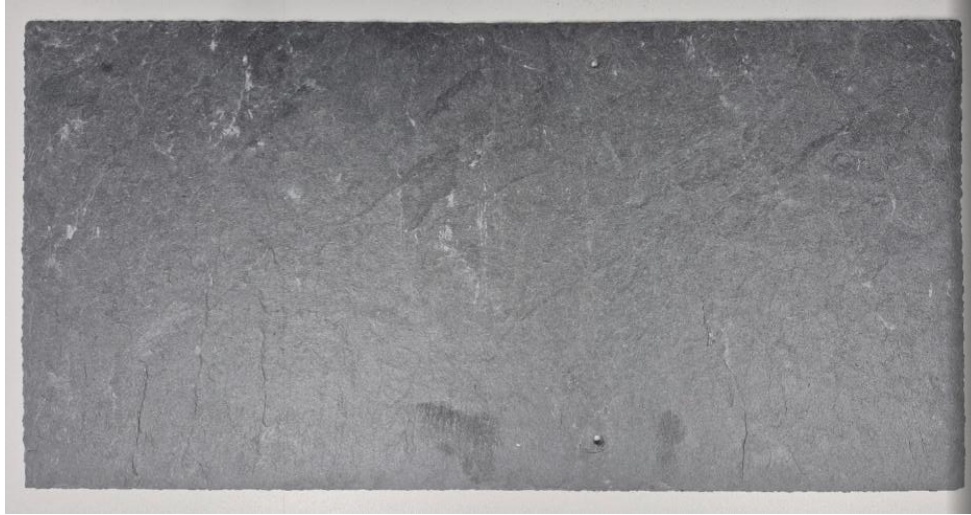
Slate sample (Garden store roof)
