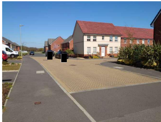
Photograph 8: Raised table arrangement on-Billy Road.
