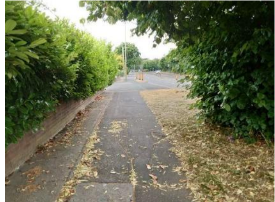
Photograph 32: Pedestrian footways along Havant Road
