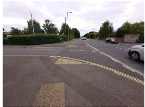
Photograph 34: Pedestrian dropped kerbs along Church Road viewing southbound
