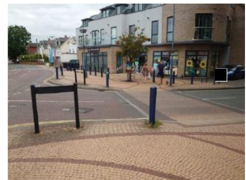
Photograph 20: West Lane/Station Road junction conditions
