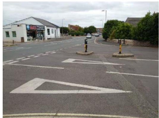
Photograph 36: St Mary's Road/Manor Road Junction pedestrian refuge island
