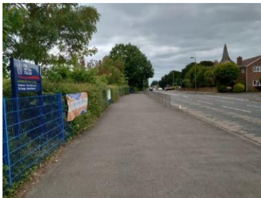
Photograph 33: Church Road pedestrian footway conditions adjacent The Hayling College viewing southbound
