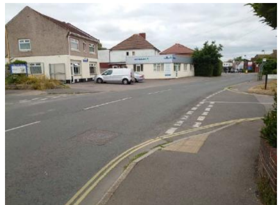
Photograph 38: Station Road pedestrian footway conditions
