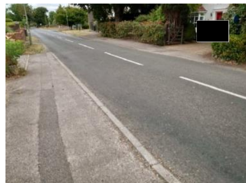
Photograph 10: West Lane dropped kerbs viewing northbound
