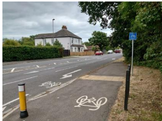
Photograph 29: Start of the cycle lane on Church Road/Manors Road roundabout
