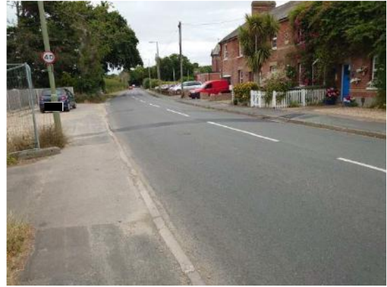
Photograph 26: Manors Road footway terminates on northbound carriageway
