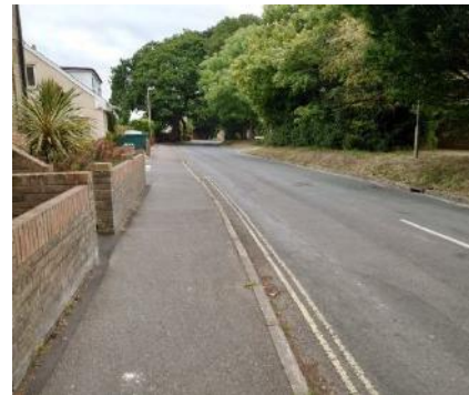
Photograph 18: West Lane conditions
