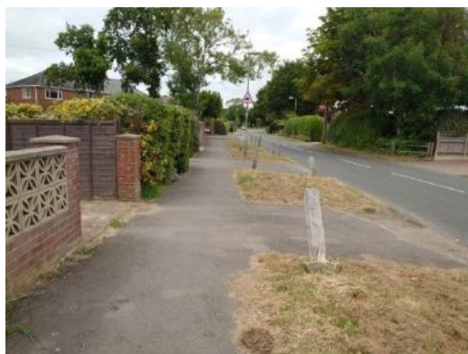
Photograph 13: West Lane conditions viewing northbound towards Saltmarsh Junction
