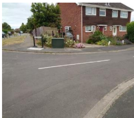
Photograph 14: Dropped Kerbs at Glebe Close/West Lane
