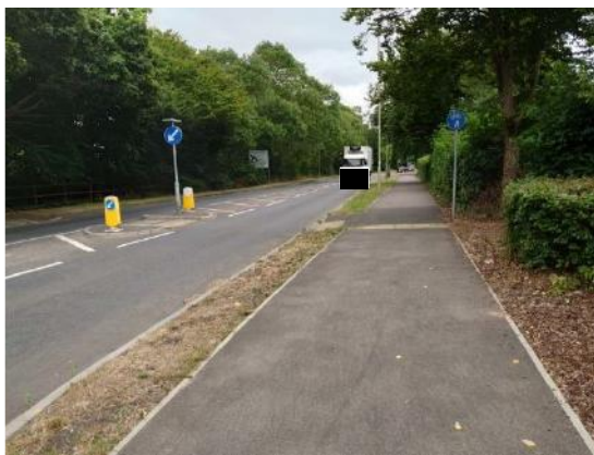
Photograph 27: Pedestrian refuge island crossing Manors Road viewing eastbound
