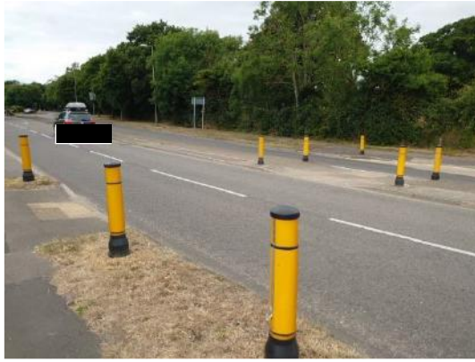
Photograph 31: Pedestrian crossings along Havant Road east of the roundabout
