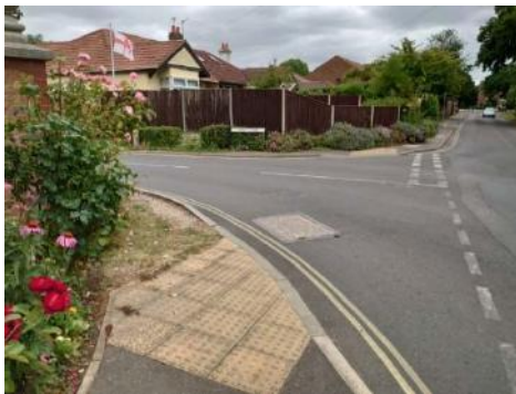
Photograph 17: West Lane tactile paving at West Lane/Newtown Lane junction
