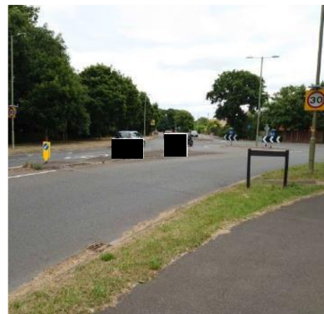
Photograph 28: Pedestrian dropped kerbs and refuge island at roundabout
