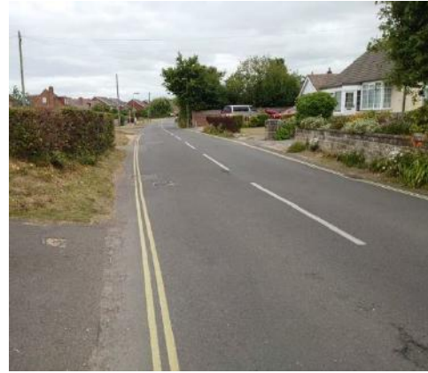
Photograph 16: West Lane conditions
