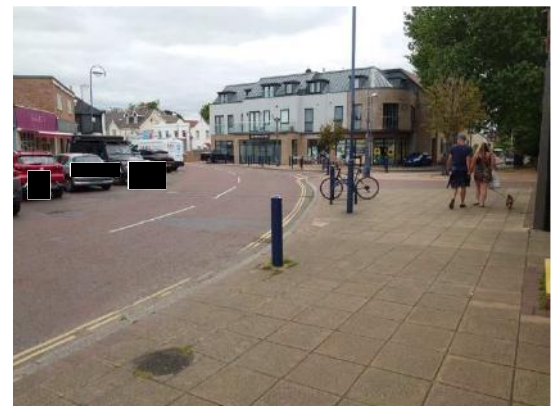
Photograph 40: Station Road pedestrian footway flush with carriageway
