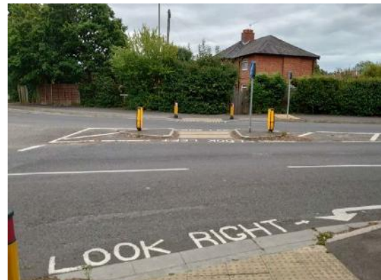
Photograph 30: Pedestrian dropped kerbs and refuge island at roundabout crossing (Church Road)
