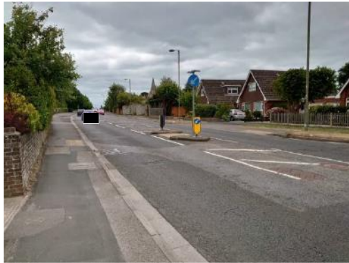
Photograph 33: Church Road pedestrian refuge viewing southbound
