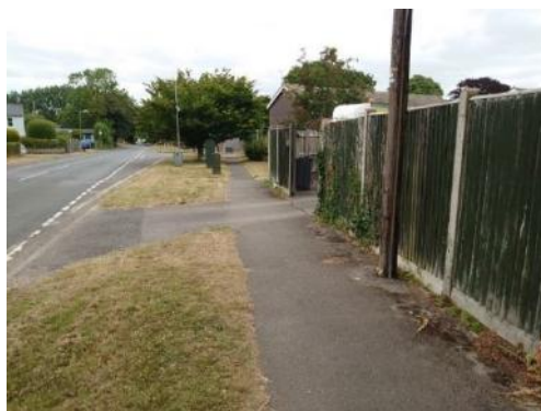
Photograph 12: West Lane pedestrian conditions viewing northbound
