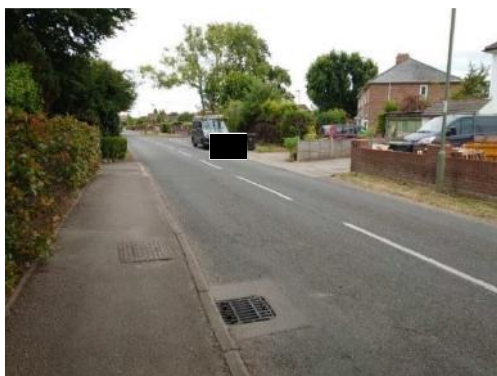
Photograph 11: West Lane conditions viewing southbound
