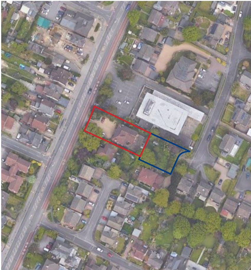
Google Maps image of application site
