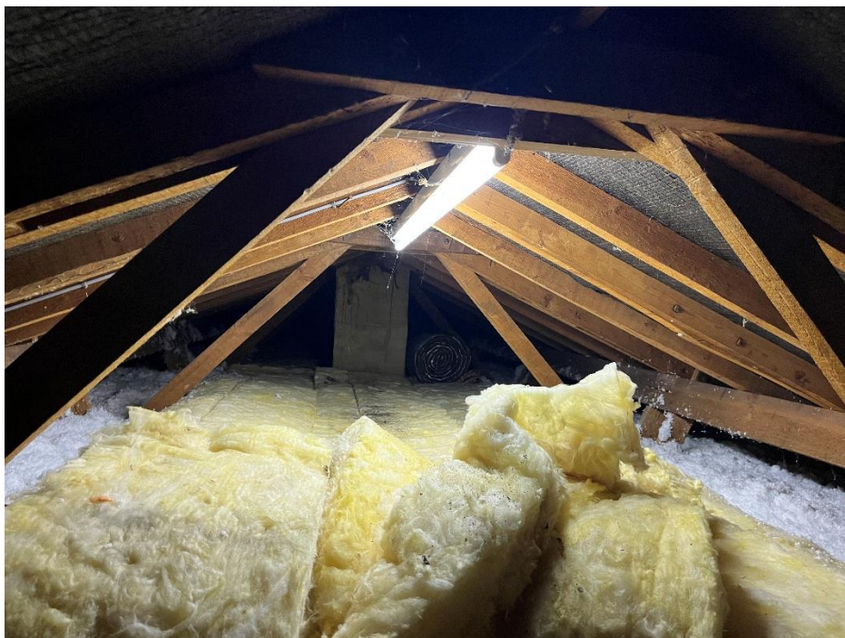
Figure 7. Main loft looking southwest
