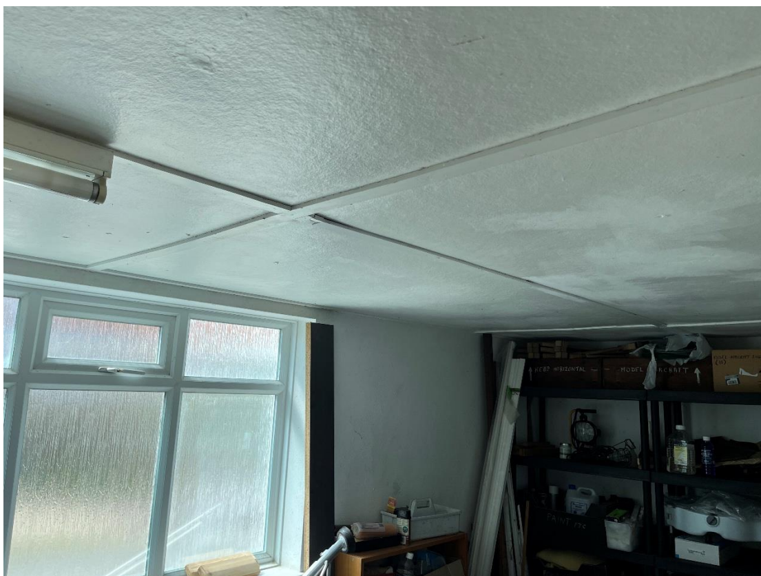
Figure 9. Interior of double garage looking northwest.
