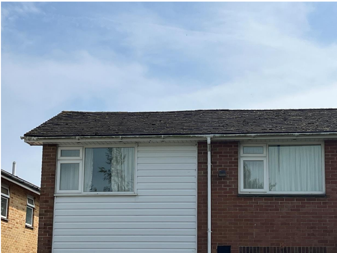
Figure 5. Rear elevations (eastern half) looking southeast.
