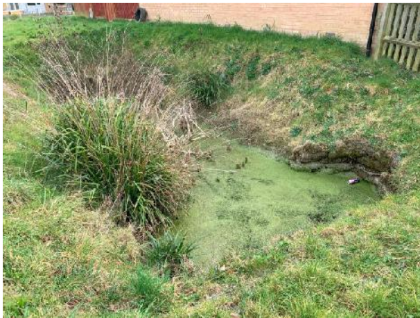
Photograph 4.8: Balancing Pond P1 connected to Ditch D1 via a culvert, east of the Site boundary
