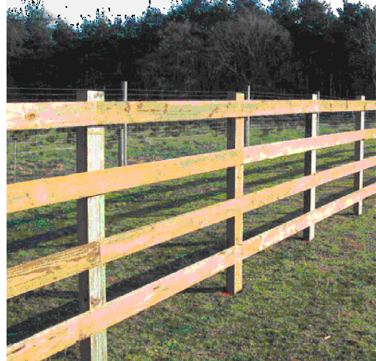
Timber Post and Rail Fence in Line with HCC specification.
