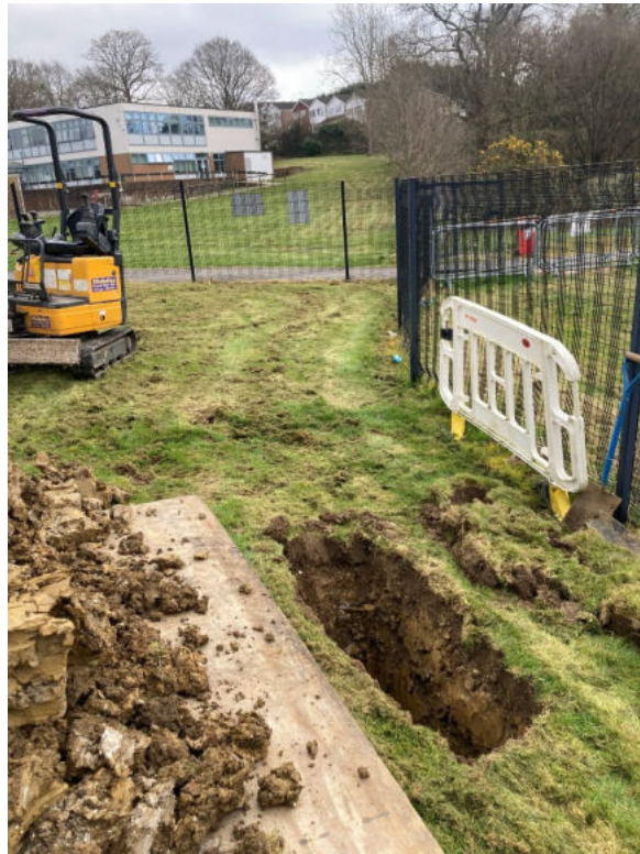
Photograph 1 : TP1 Excavation Location
