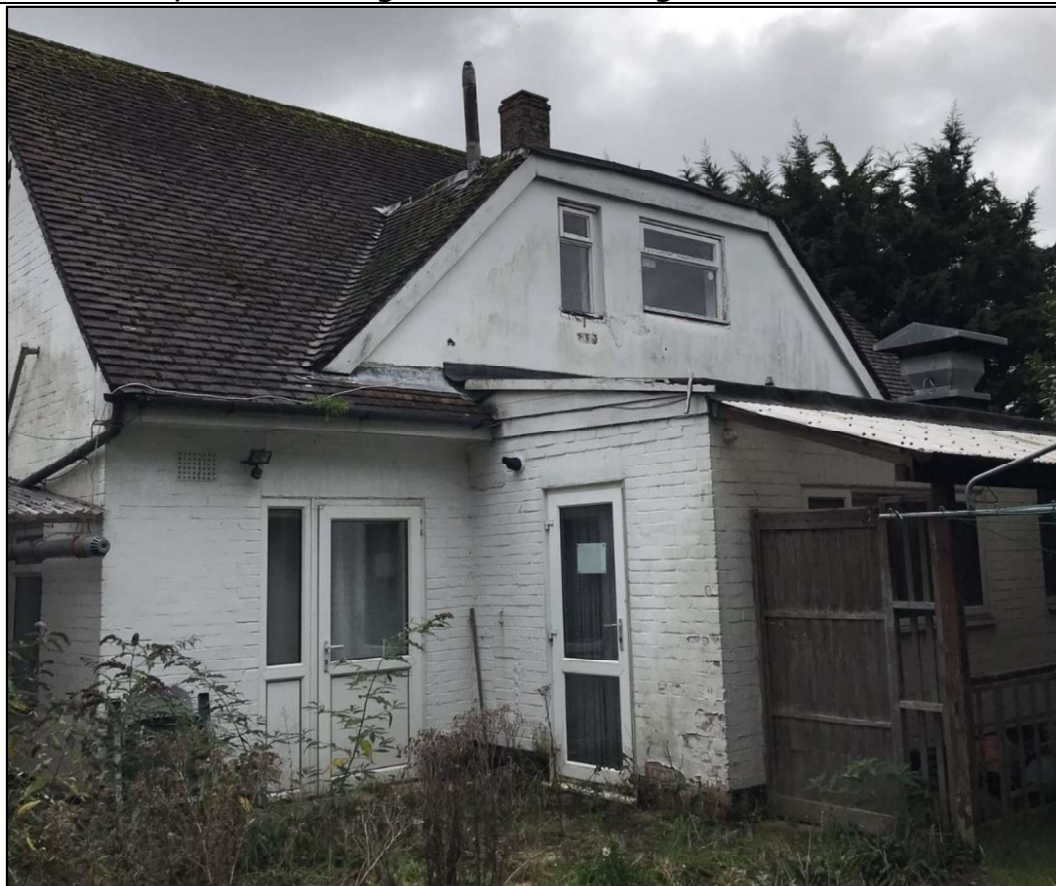
Photo 4: B1, main building. North-west
