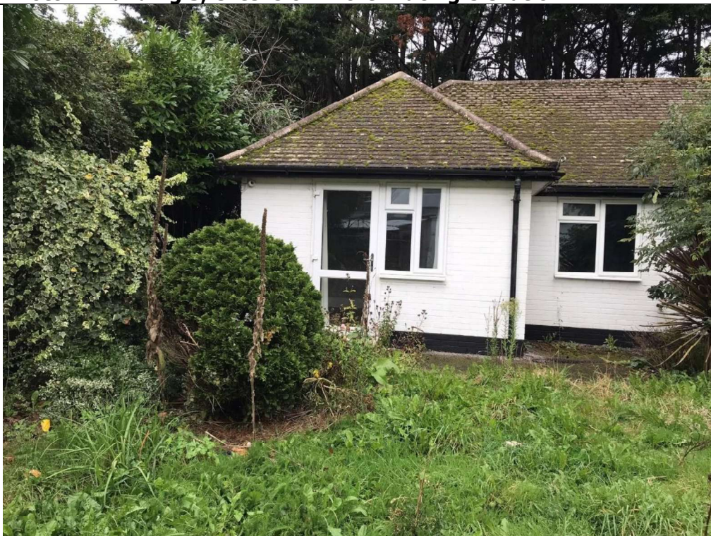
Photo 2: Building 3, extension. South-facing elevation
