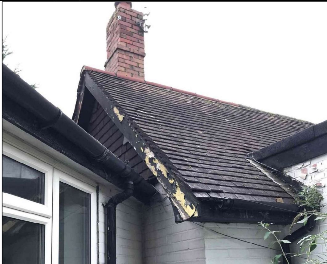
Photo 6: B2, reception building
