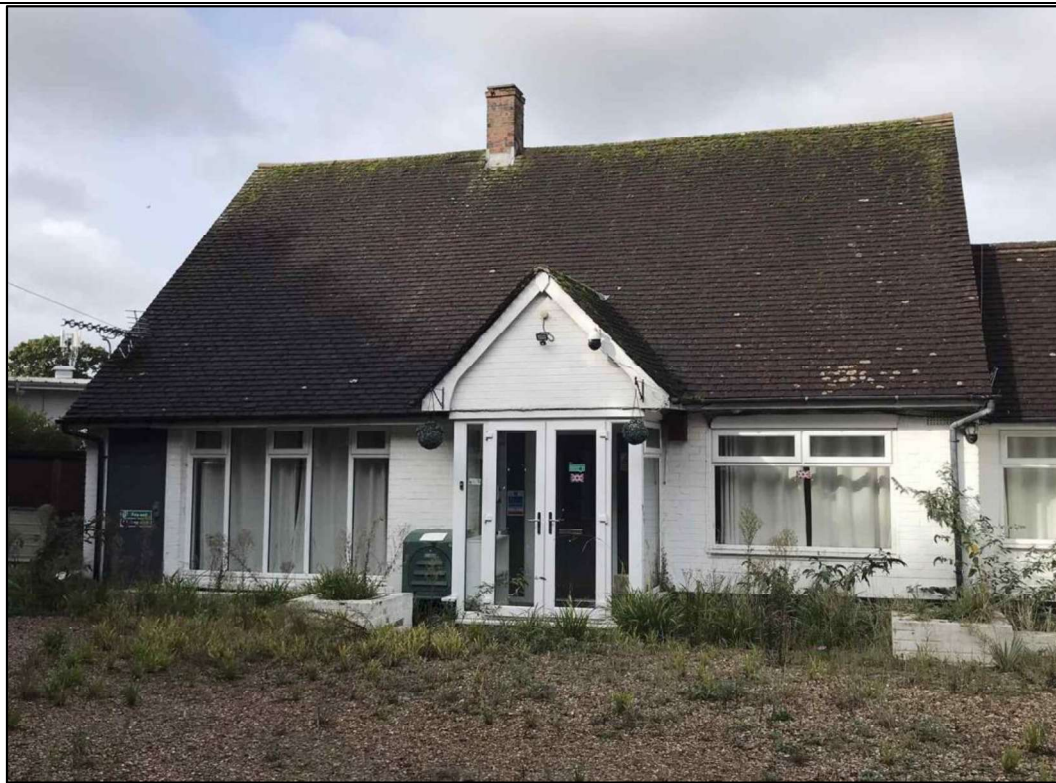
Photo 3: B1, main building. South-east facing elevation
