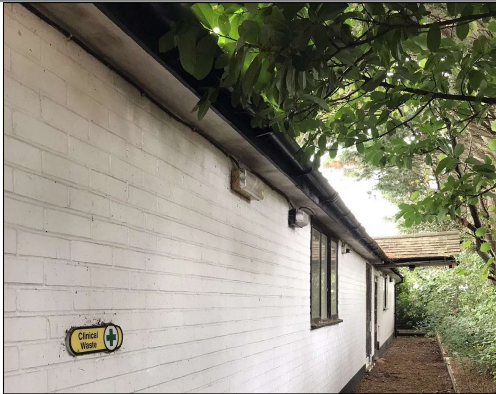
Photo 1: Building 3, extension. North-facing elevation
