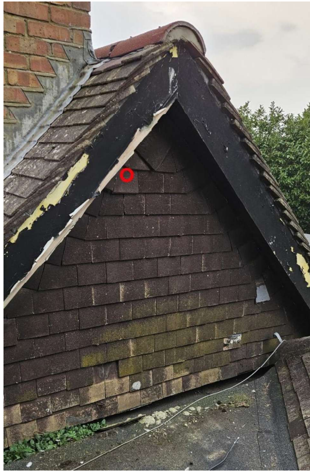
Photo 1 – Location of Common Pipistrelle under hanging tiles of the east gable end of building 2 (B2)
