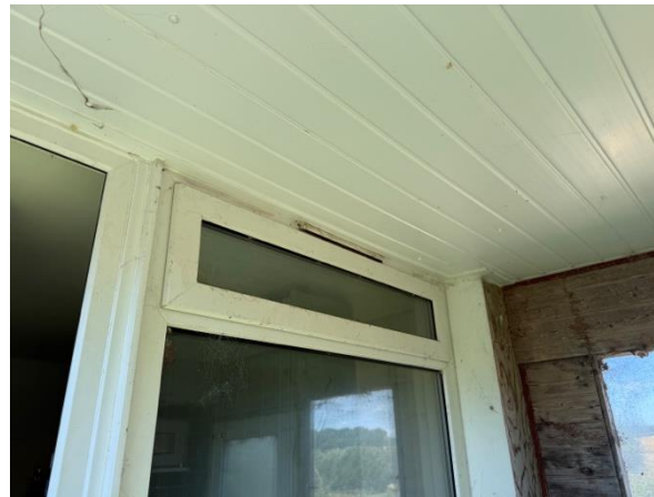
Existing windows and doors condition
