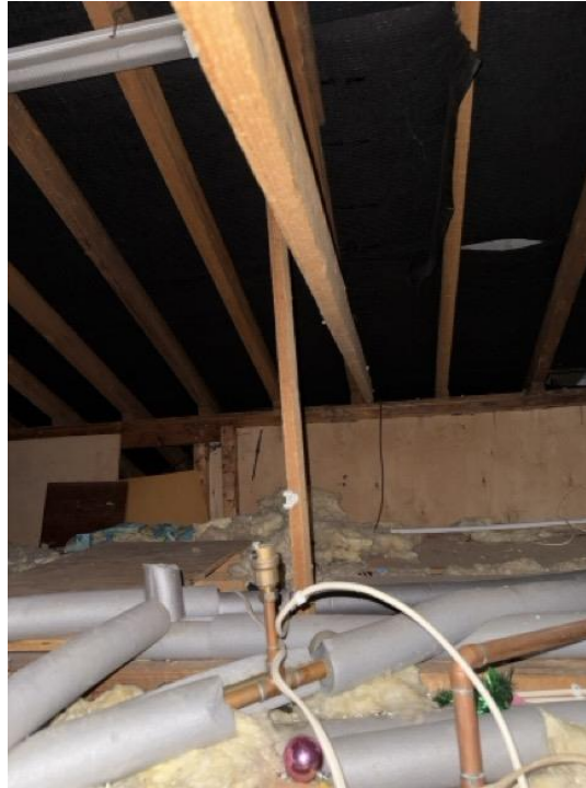
Existing loft insulation
