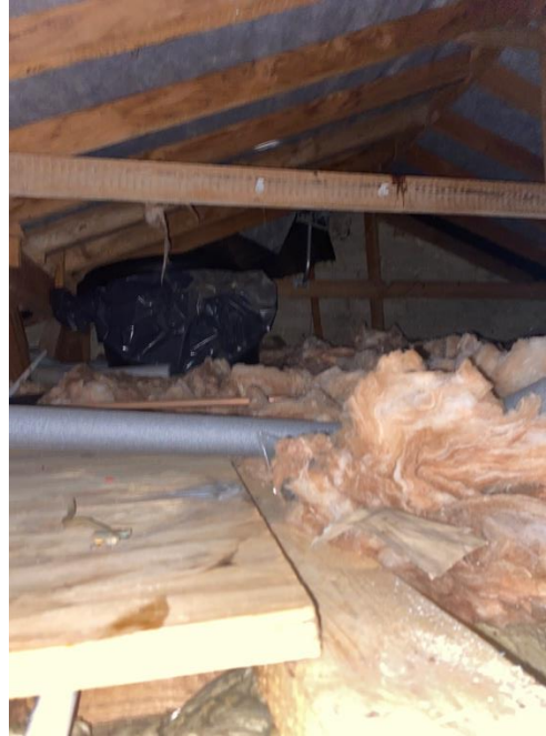
Existing loft insulation
