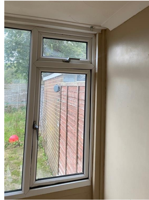
Rear garden and timber fence
