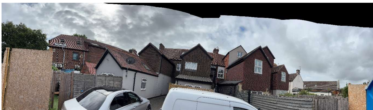
Panoramic view of the rear (north) elevations of nos.64-80 West Street, viewed from the north on the subject site.
