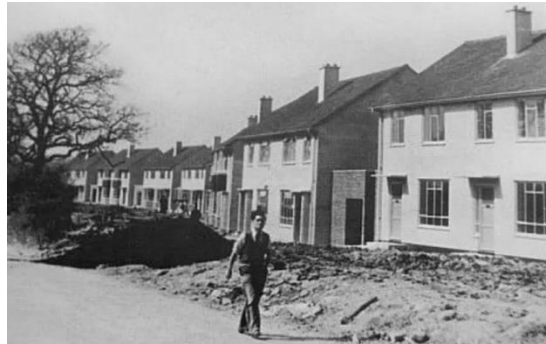
Above left: Construction of post-war housing in Leigh Park in the 1950s
