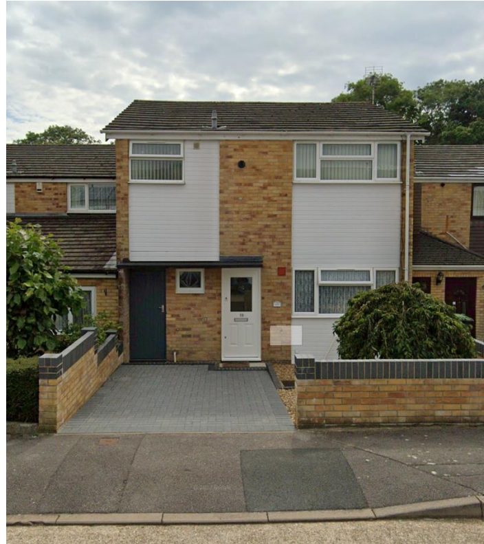
Existing external front elevation
