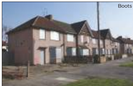
■ Examples of timber framed properties before refurbishment
