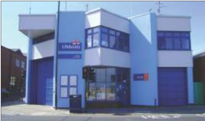
■ Redcar Lifeboat Station now benefits from an External Wall Insulation system with a silicone finish
