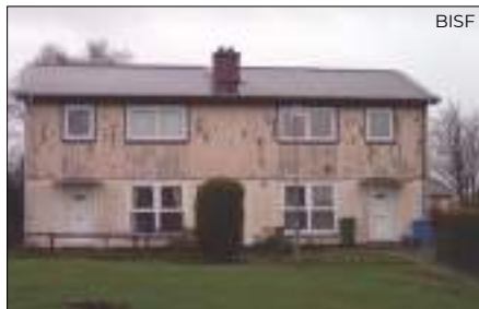
■ Examples of metal framed properties before refurbishment
