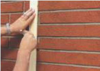
■ Photograph Notes: Cutting through top coat to reveal the mortar Layer.
