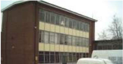
■ Kesteven & Grantham Girls School Before Refurbishment
