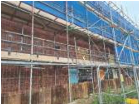
■ Goffs Academy during construction
