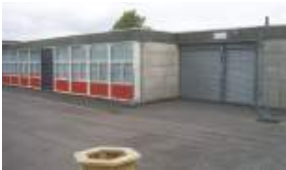
■ Chryston Primary School, Glasgow CLASP System built school with failing concrete Cladding panels
