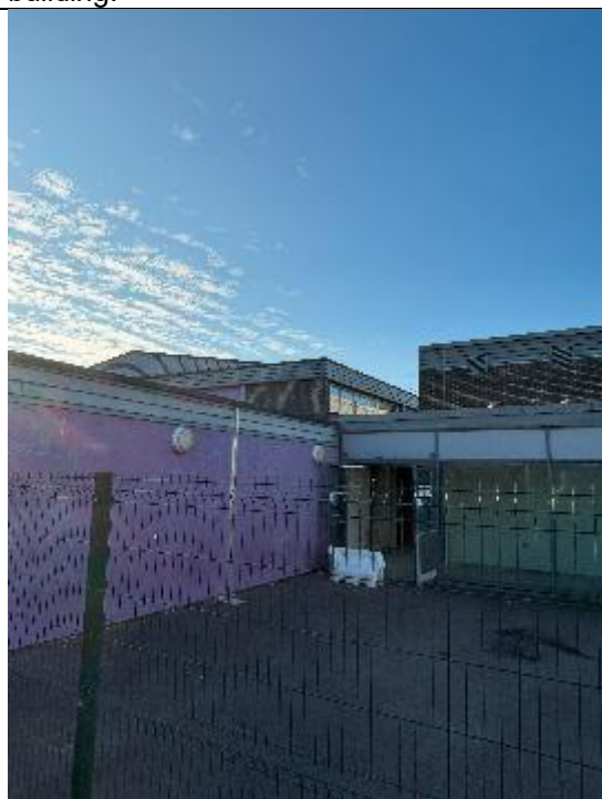
Photograph 3: North facing elevation of building.
