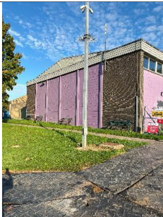
Photograph 1: View of South facing elevation of building.
