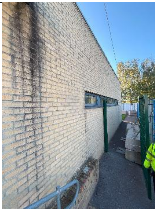
Photograph 4: West facing elevation of building.
