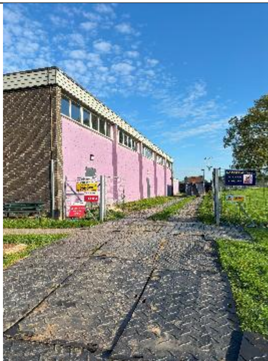
Photograph 2: View of East facing elevation of building.
