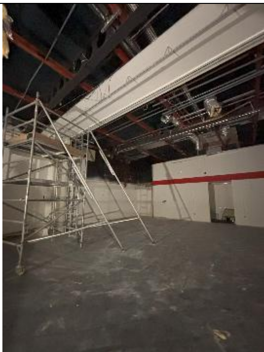
Photograph 5: View of internal inspection ceiling. Material to be stored within the building.
