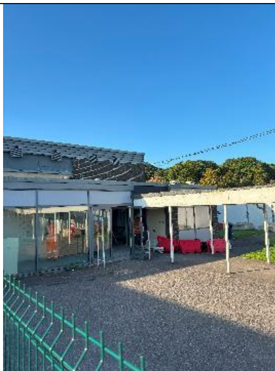
Photograph 10: View of northwestern area of the building subject to demolition.
