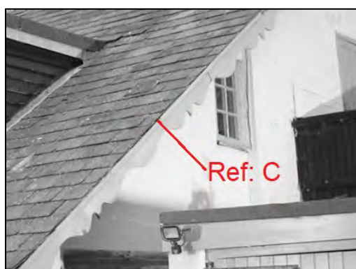
Figure 48: Access feature C, upon the western gable end
