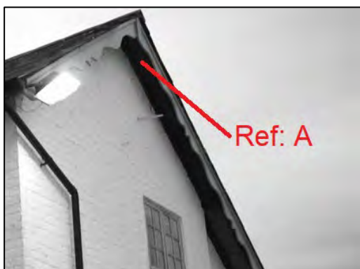
Figure 46: Access feature A, at the apex of the eastern gable end
