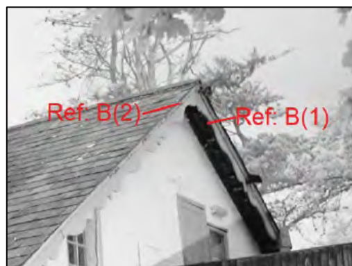
Figure 47: Access features B(1) and B(2), upon the western gable end
