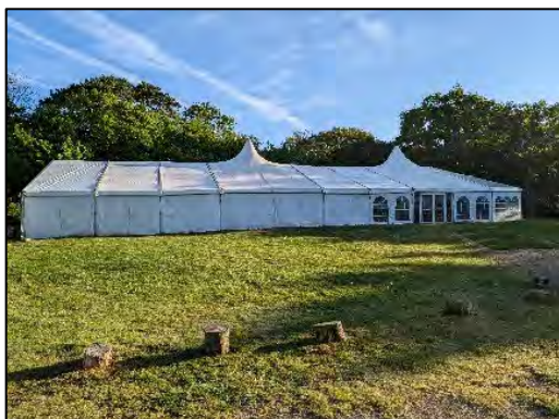
Figure 23: Northern elevation of marquee
