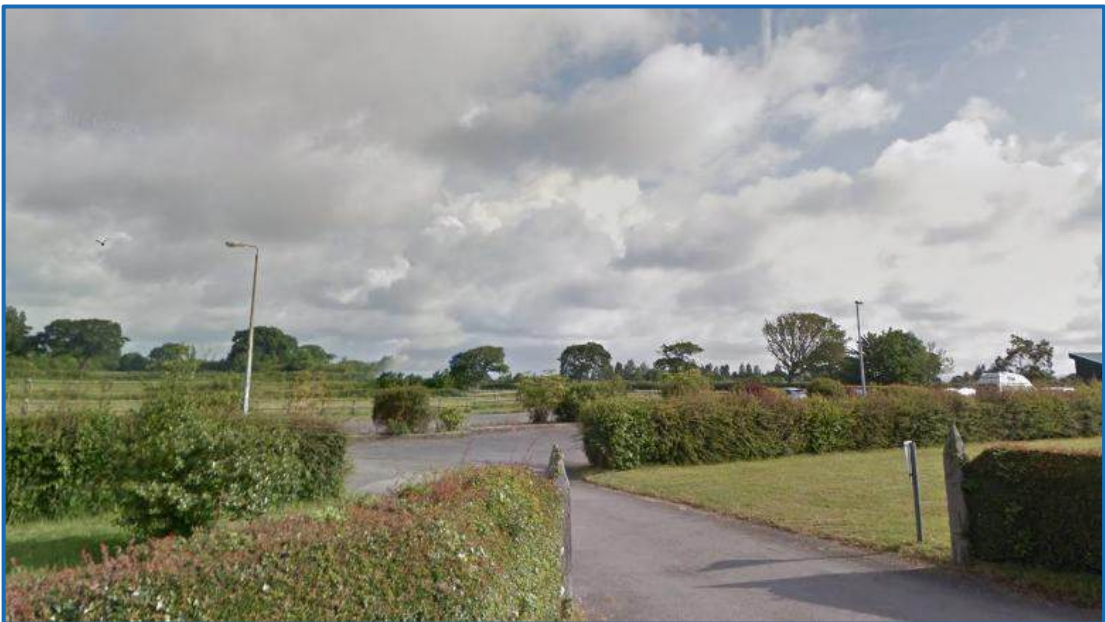
Figure 4: View of the Existing Lighting Associated with the Car Park for Coffee on the Green Hayling
