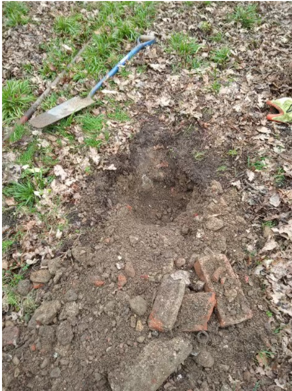
Photo 2: Hand dug trial hole
