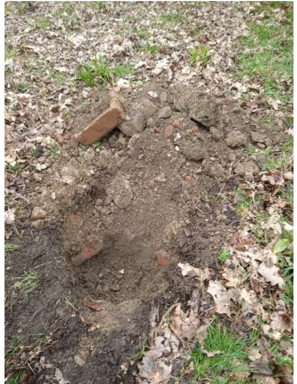
Photo 3: Trial hole showing rubble and old bricks beneath surface of track.
