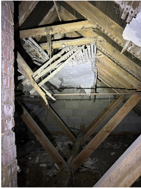
Image 9. A view of the loft in the two-storey section of the dwelling.
