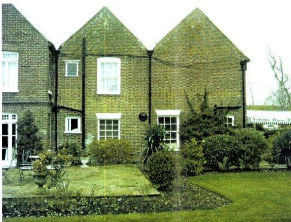
2.2 Terrace and adjoining windows to office and WCs.
