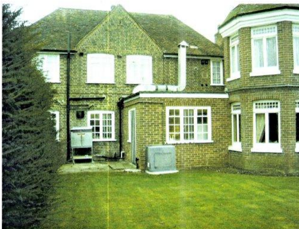
2.4 Kitchen area adjacent to restaurant
