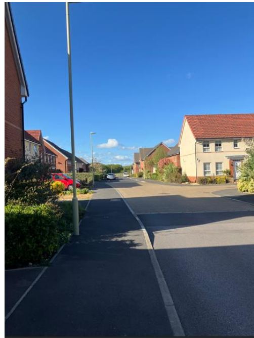
Photograph 2: Conditions on Billy Road south of Signal Way
