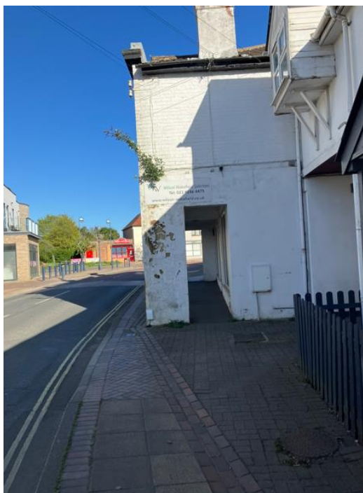
Photograph 9: Existing footway narrowing along Station Road
