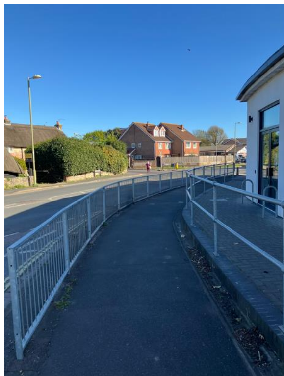
Photograph 17: Railings present along the eastern side of junction with Manor Road
