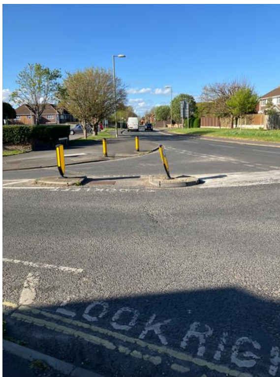
Photograph 16: Pedestrian facilities present at junction with Manor Road
