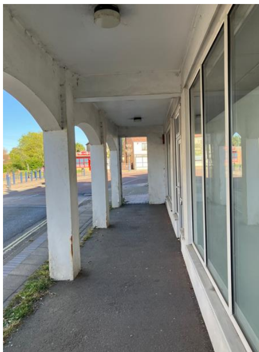
Photograph 10: Alternative wider route through existing building
