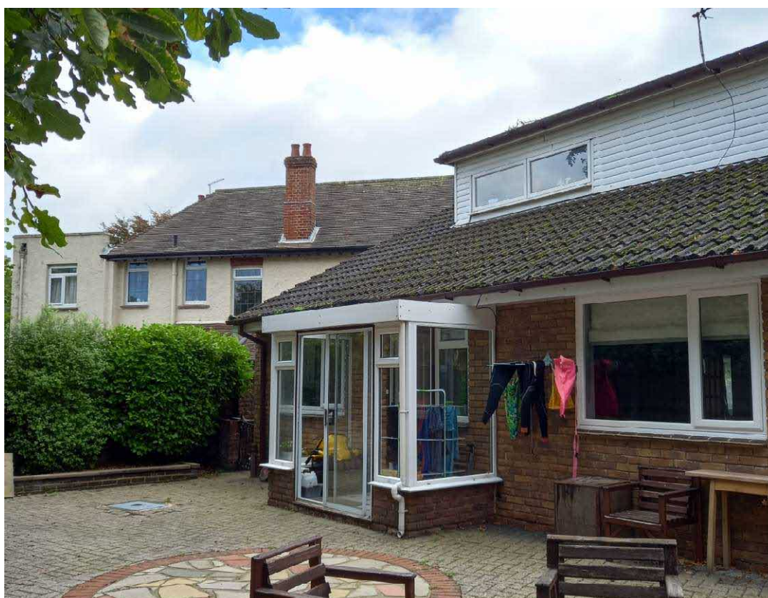
Rear elevation looking south-east.
