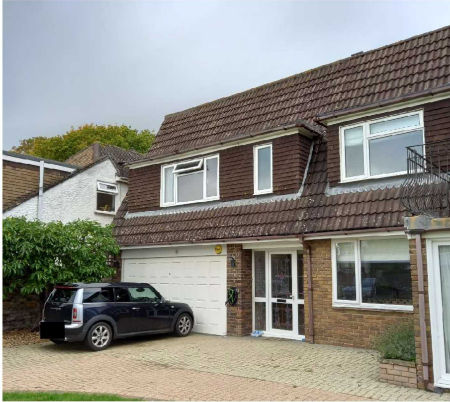
Front elevation looking north-west.
