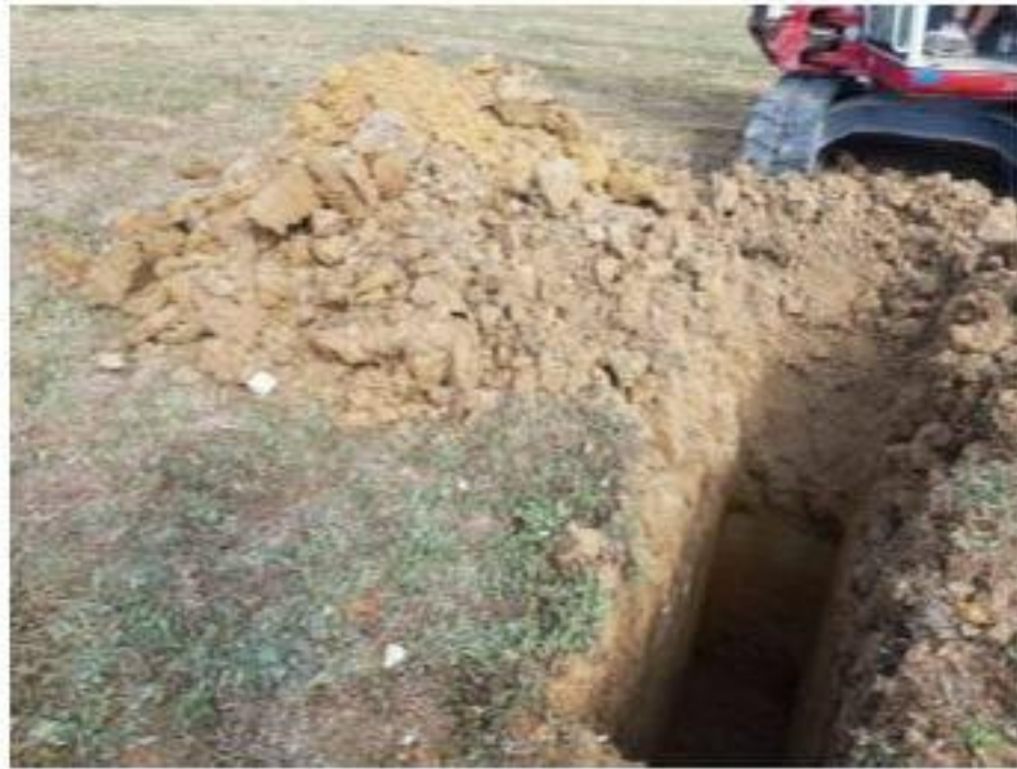
PLATE 05 – Overview of TP10 in parcel 3b.
