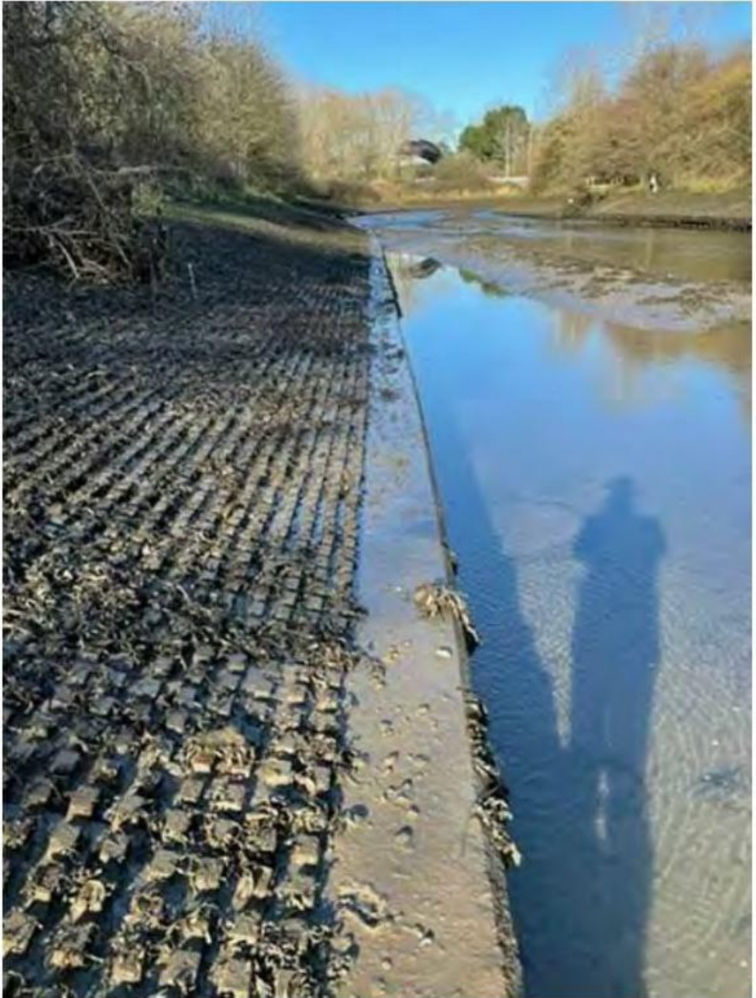
Photograph 9 – Concrete Headworks Structure Above Sheet Pile Wall (Client Provided)
