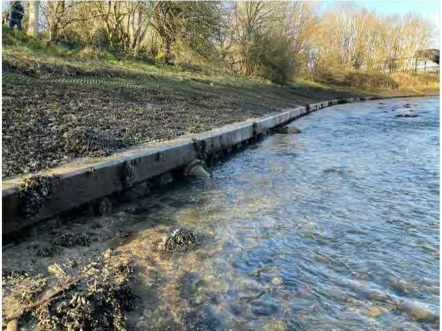
Photograph 10 – Sheet Pile Wall (Client Provided)
