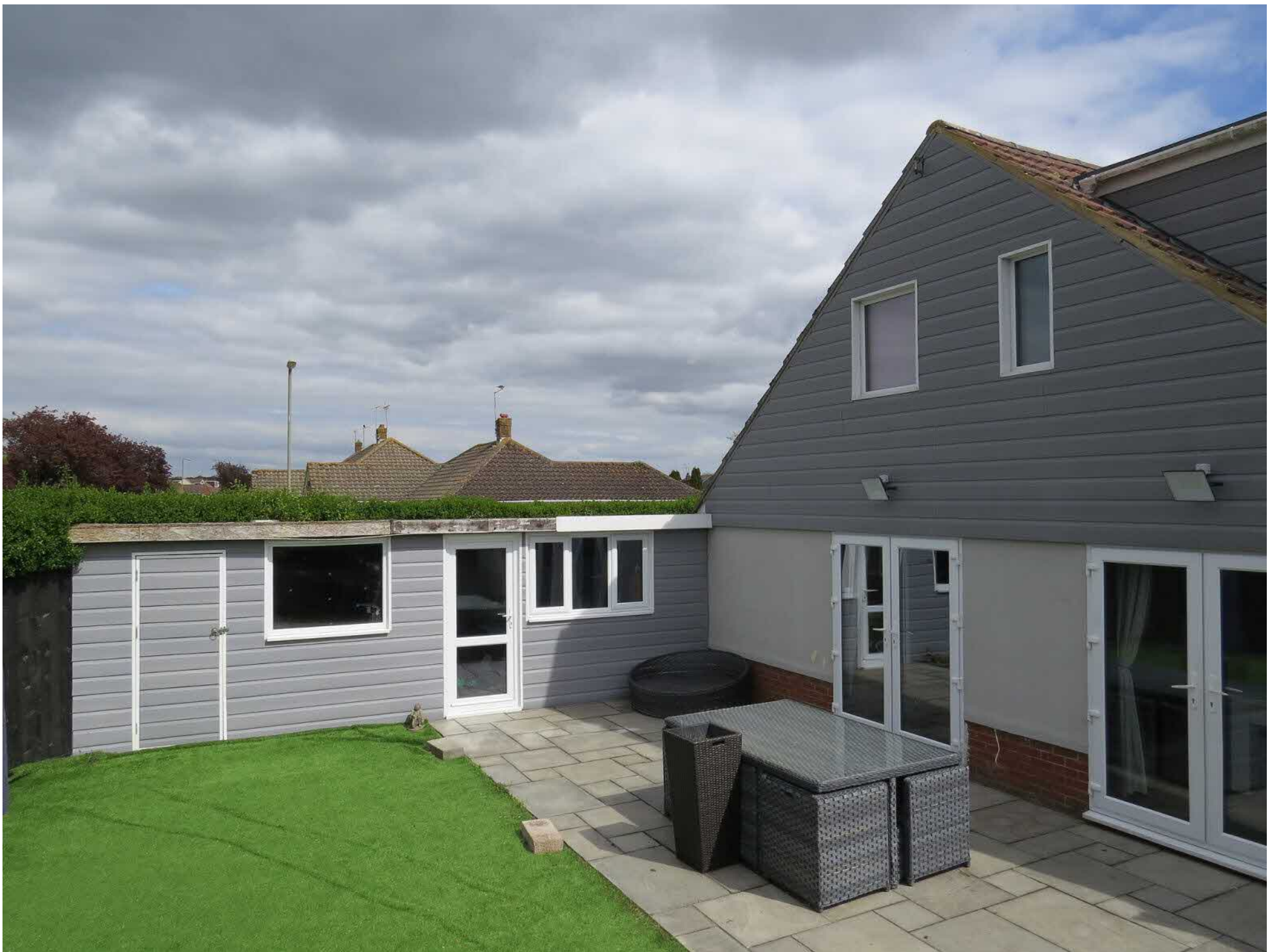
08_IMG_0985_West Facade and Outbuilding from Garden
