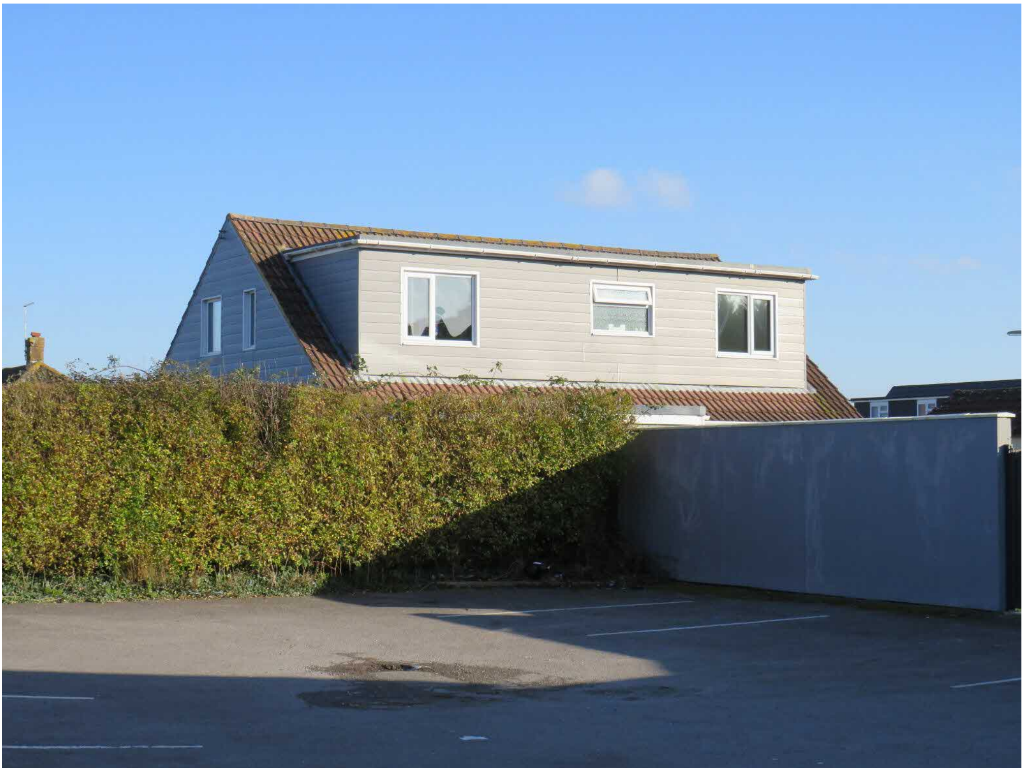
03_IMG_0411_61 Esher Grove South and West Facades
