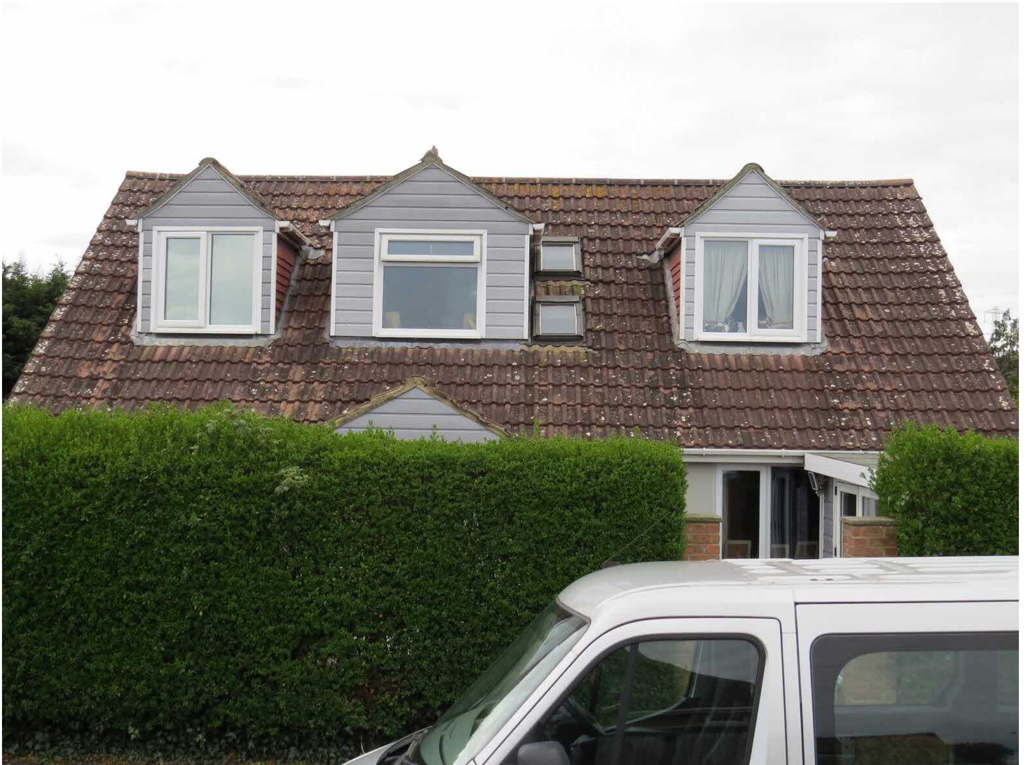
11_IMG_1094_North Facade Obscured by Hedge
