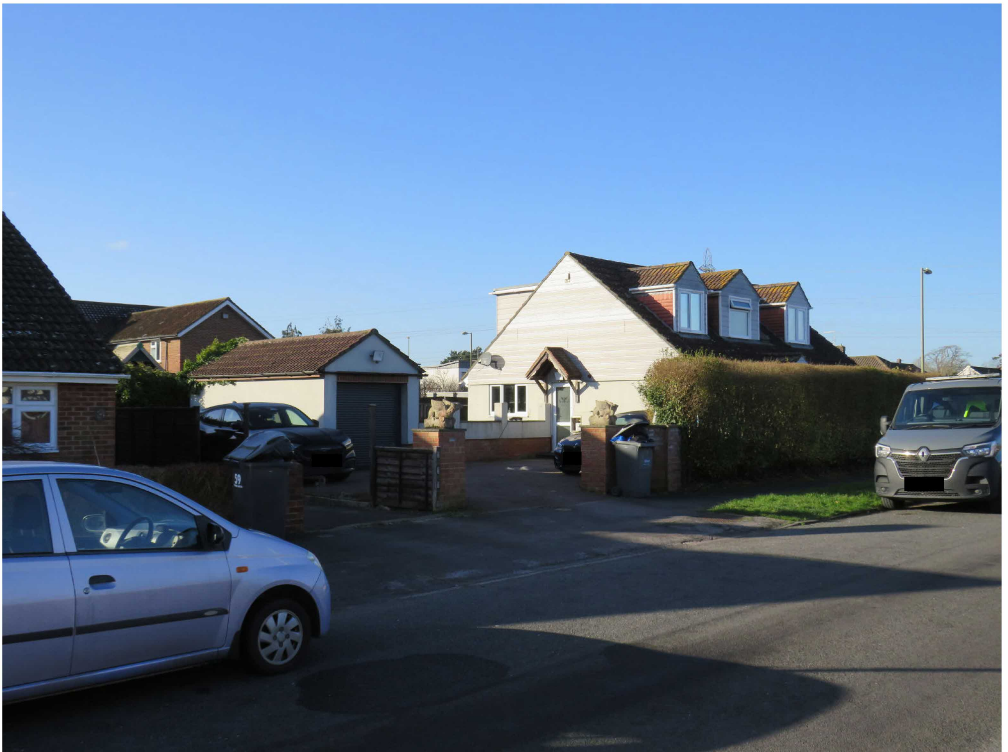
04_IMG_0416_61 Esher Grove North and East Facades
