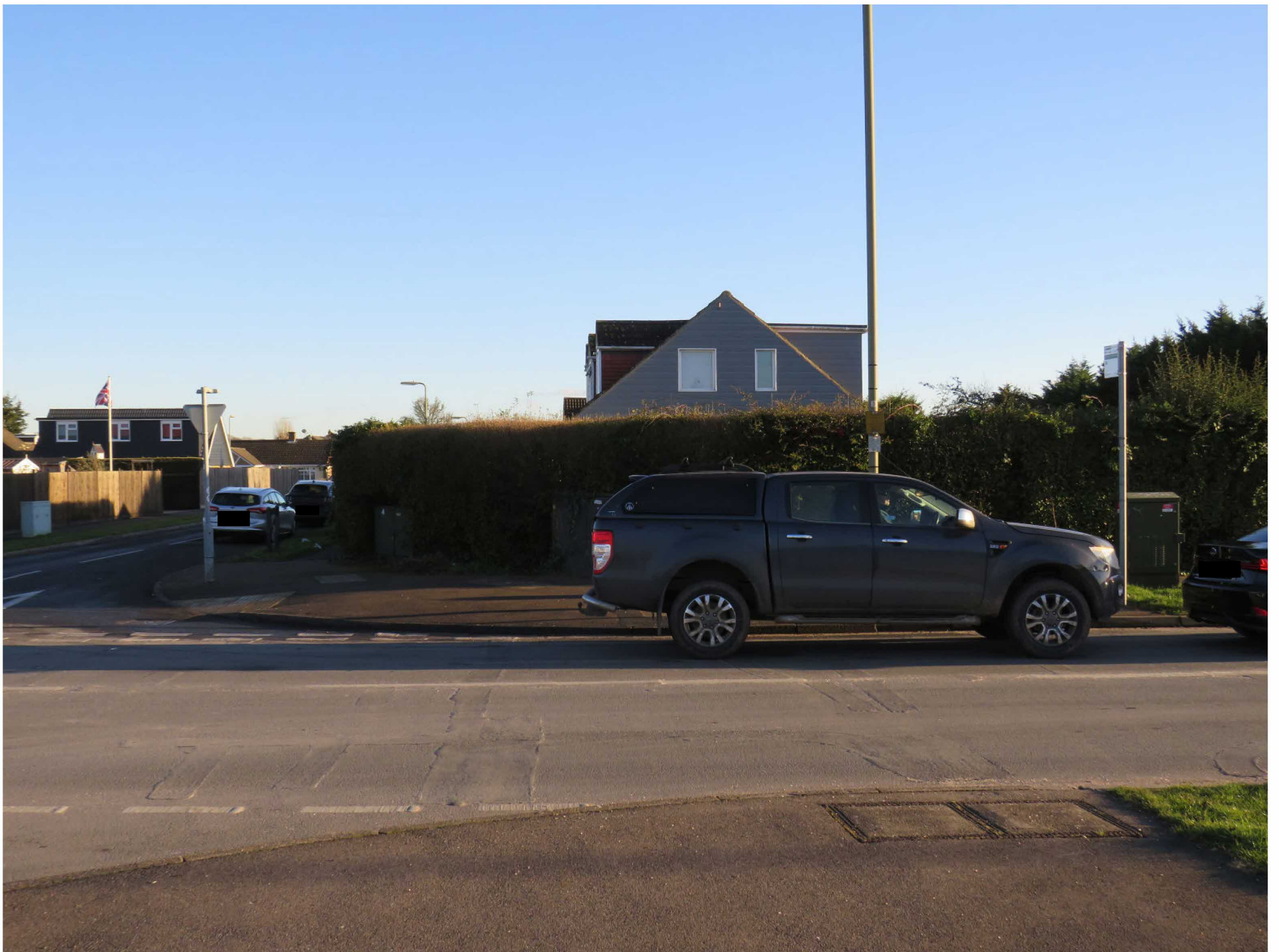
07_IMG_0493_61 Esher Grove West Facade
