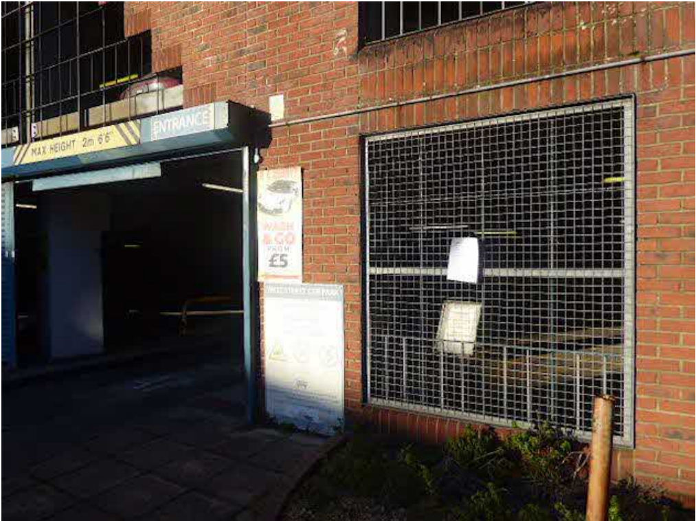
Photograph 2 – Further view of the Notice on the south elevation.
