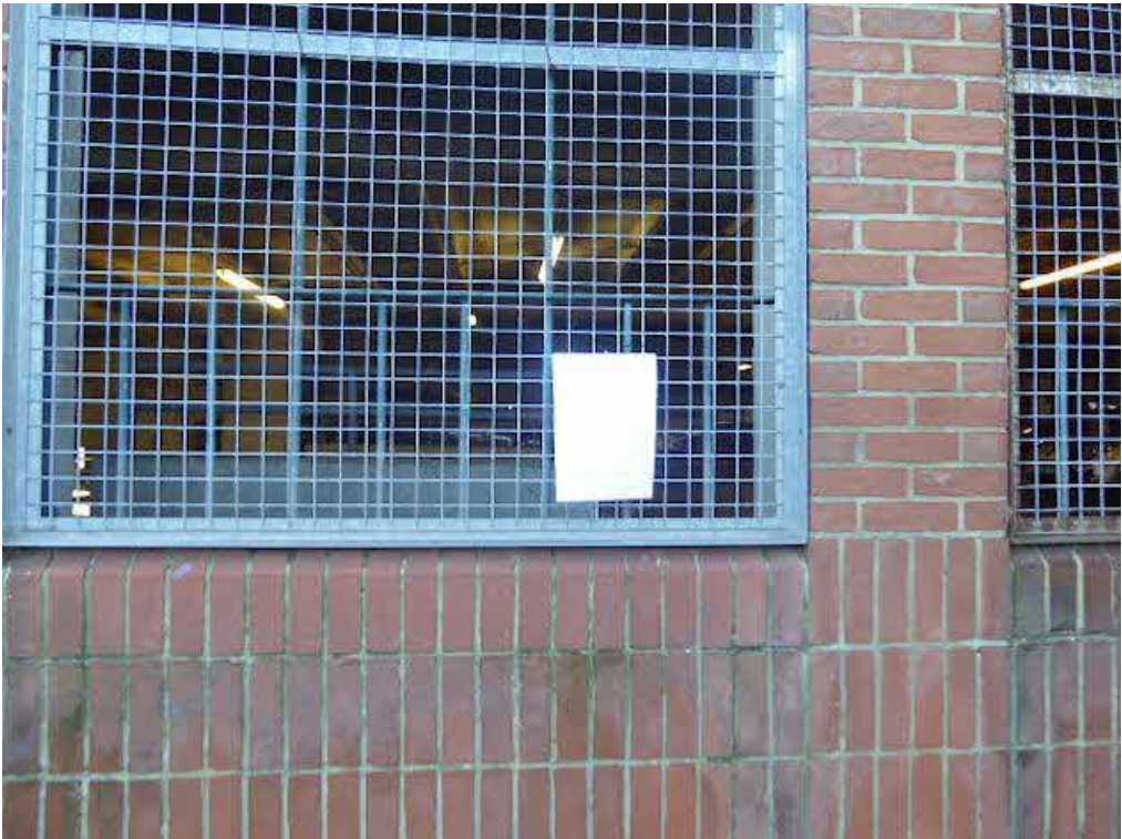
Photograph 5 – Further view of the Notice on the east elevation.
