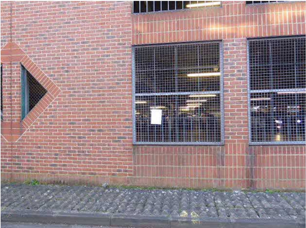
Photograph 7 – View of the notice on the north elevation.
