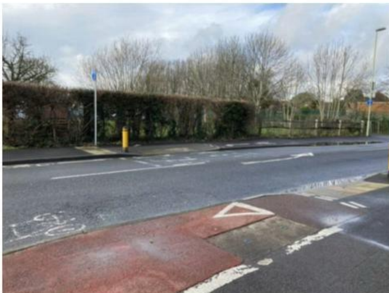
Photograph 3: Pedestrian Crossing on Southleigh Road
