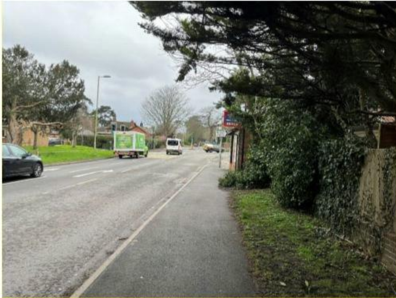
Photograph 18: Continuation of footway on Emsworth Rd
