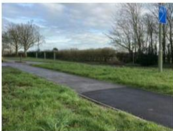
Photograph 10: Footway along Havant Road
