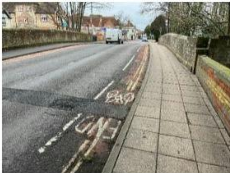
Photograph 24: East St visibility and on street cycle provision looking west
