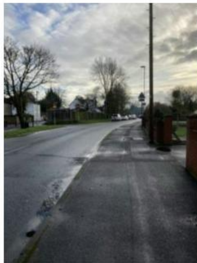
Photograph 2: Footway on Southleigh Road (towards Emsworth Road)
