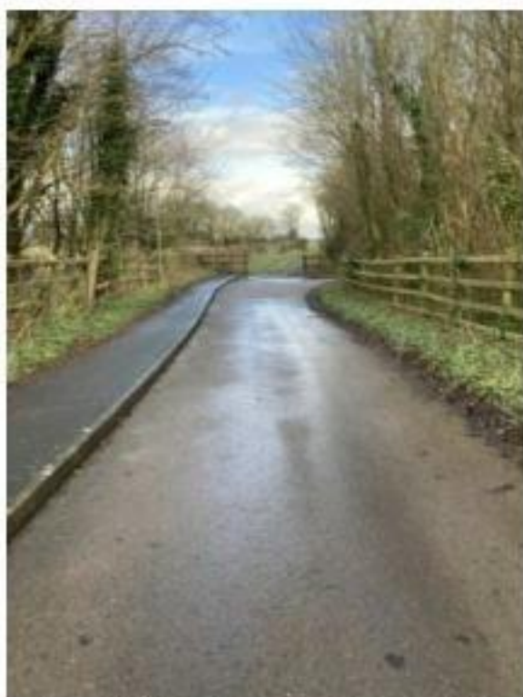
Photograph 8: Footway along Emsworth Road
