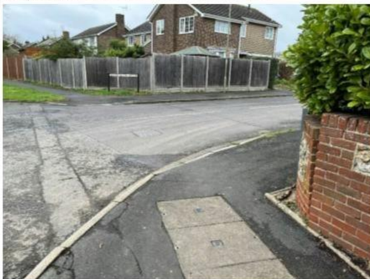
Photograph 17: Emsworth Rd / Warblington Avenue Junction
