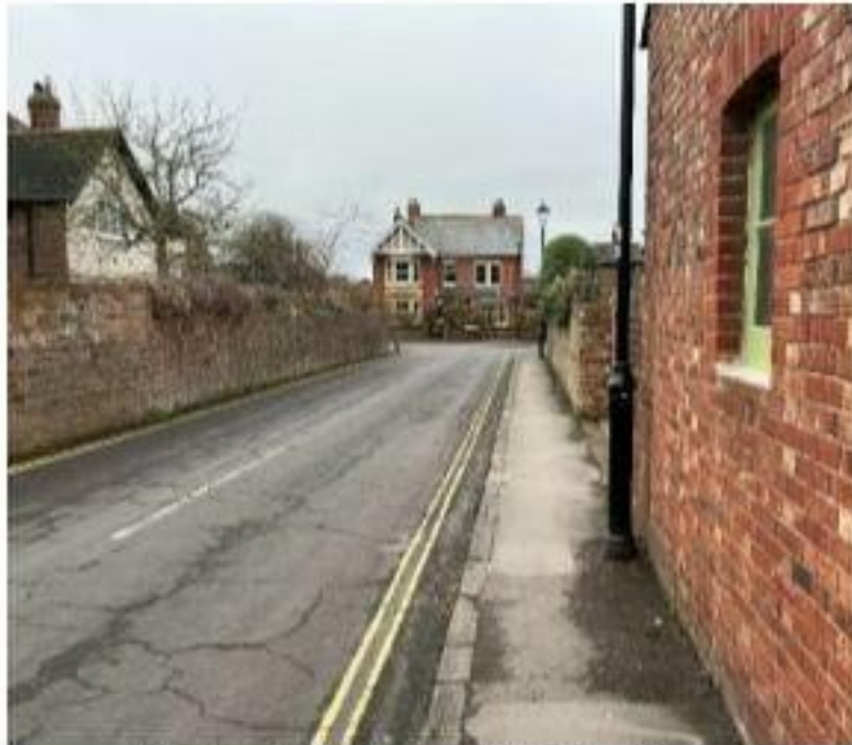
Photograph 26: Town Hall Rd Conditions
