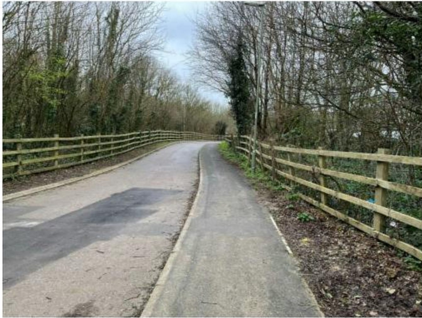
Photograph 13: Carriageway and footway conditions of Emsworth Rd
