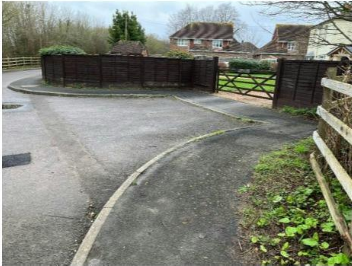
Photograph 14: Carriageway and footway conditions of Emsworth Rd
