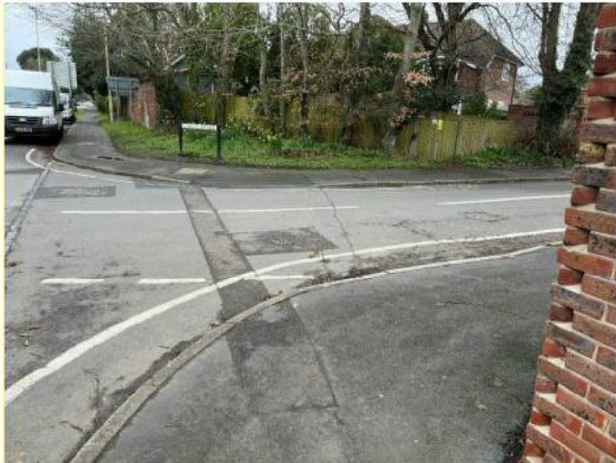
Photograph 15: Emsworth Rd / Castle Avenue Junction
