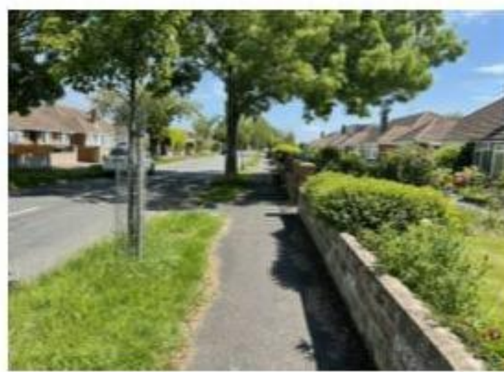
Photograph 11: Footway along Selangor Avenue
