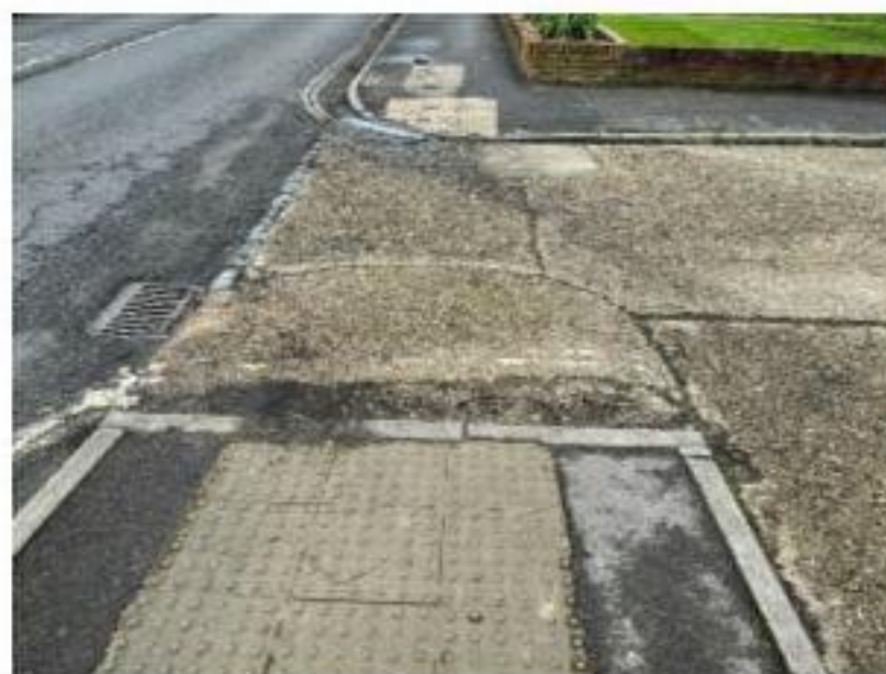
Photograph 22: dropped kerbs and tactile paving at parking layby on Emsworth Rd
