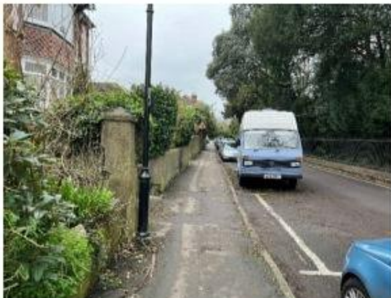
Photograph 28: South St Conditions
