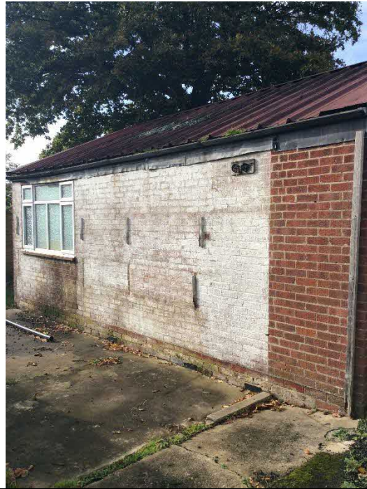
Left hand flank wall of garage
