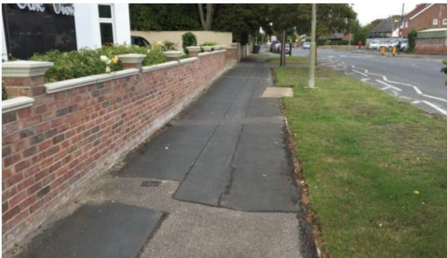
Footway Flanking Beach Road
