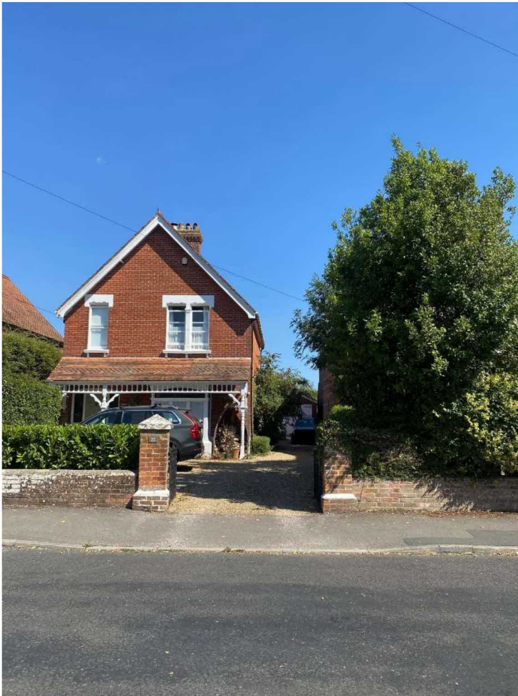
Figure 4: Front elevation photograph.
