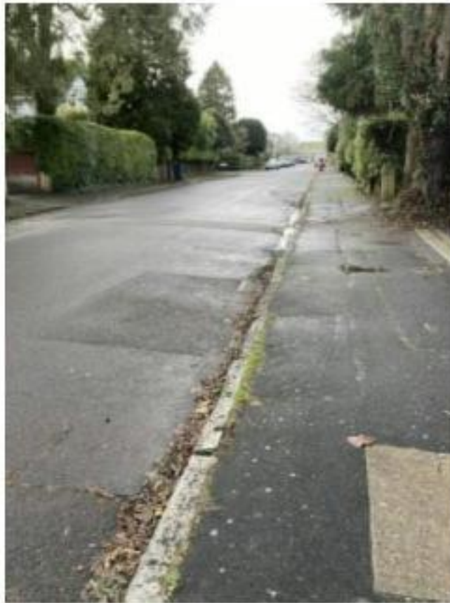
Photograph 1: Footway on St George's Avenue (towards Southleigh Road)
