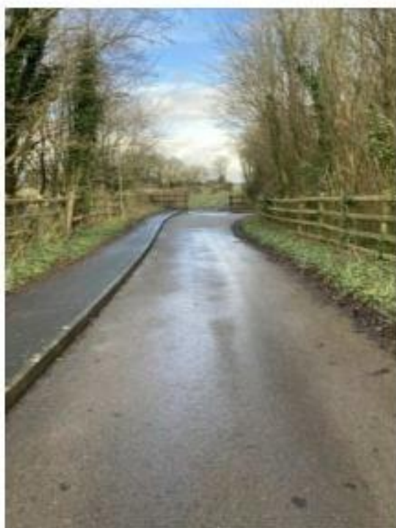
Photograph 8: Footway along Emsworth Road
