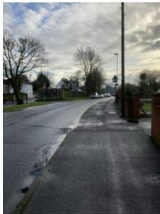
Photograph 2: Footway on Southleigh Road (towards Emsworth Road)
