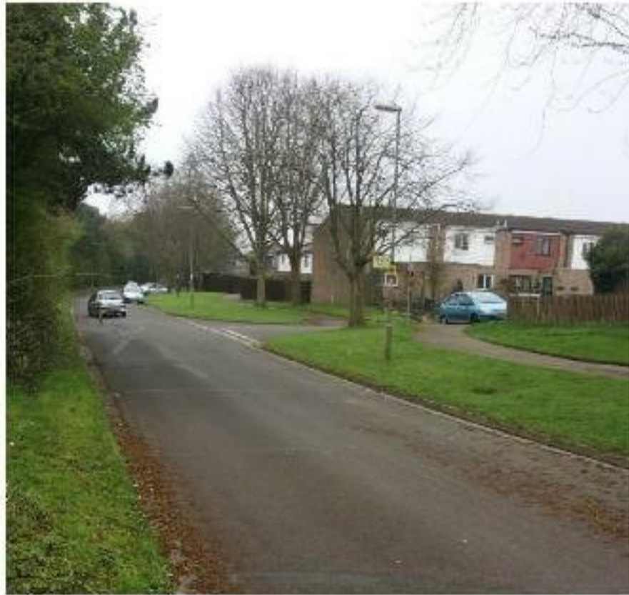
Photograph 2: Atlantis Avenue Existing Conditions
