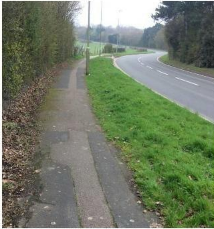
Photograph 1: Existing College Road Conditions
