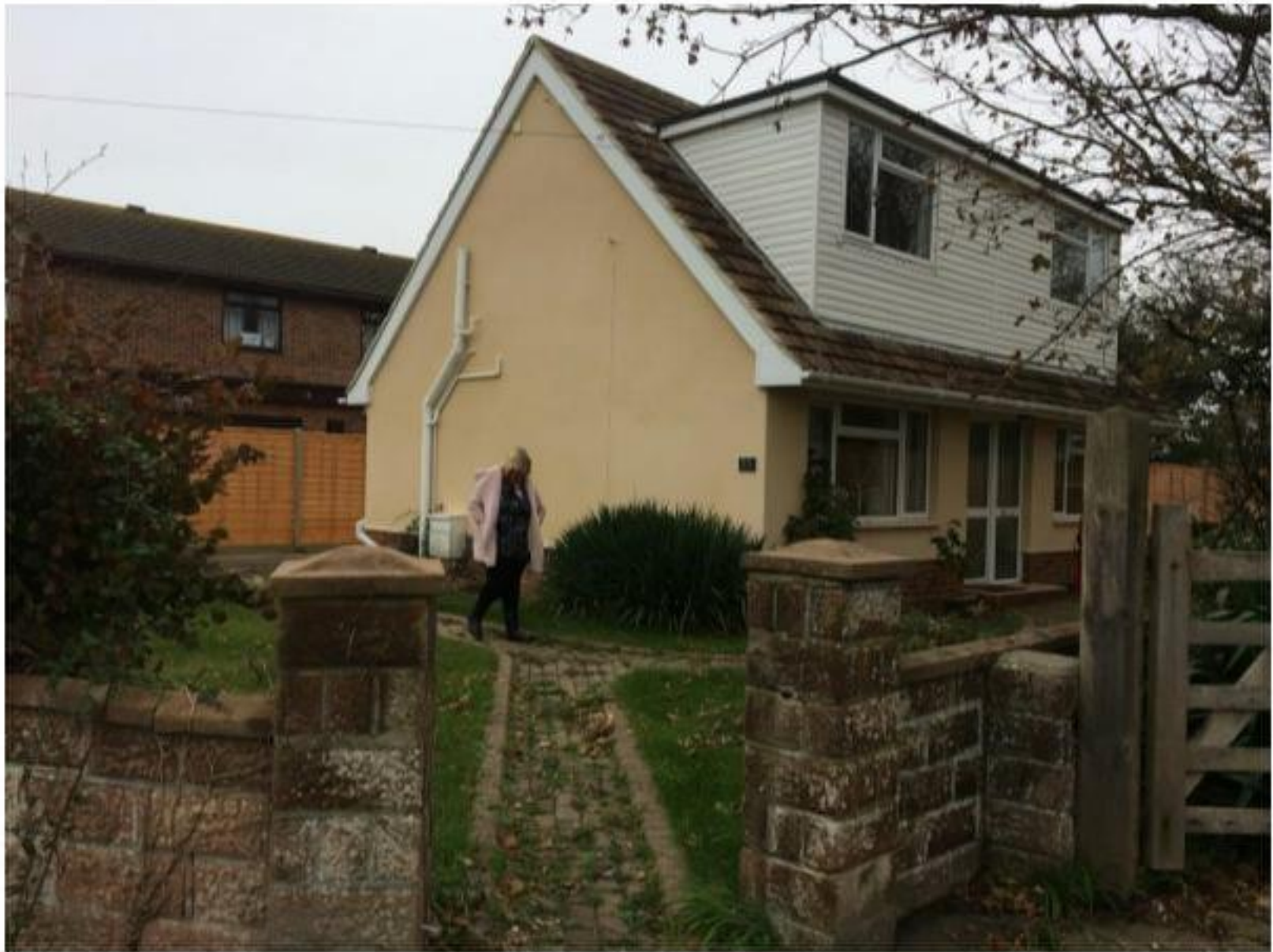
Photo 3: Front of Property
