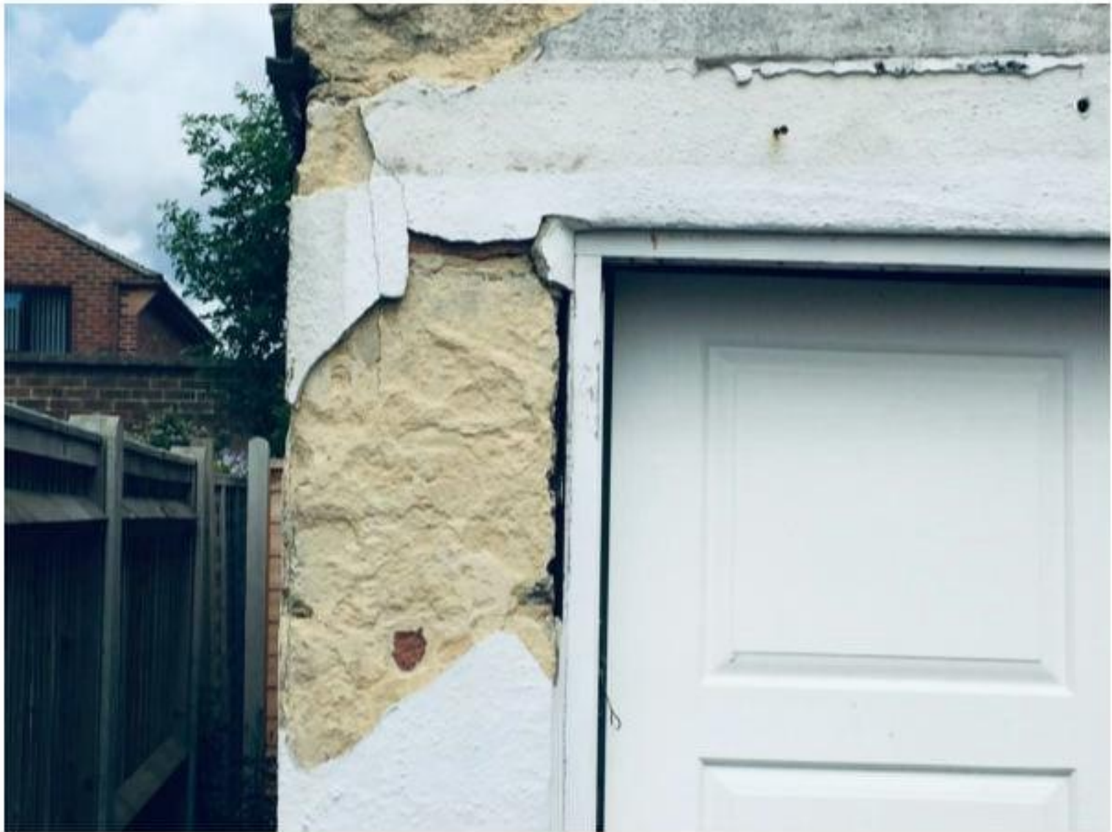
Photo 10: Side of garage
