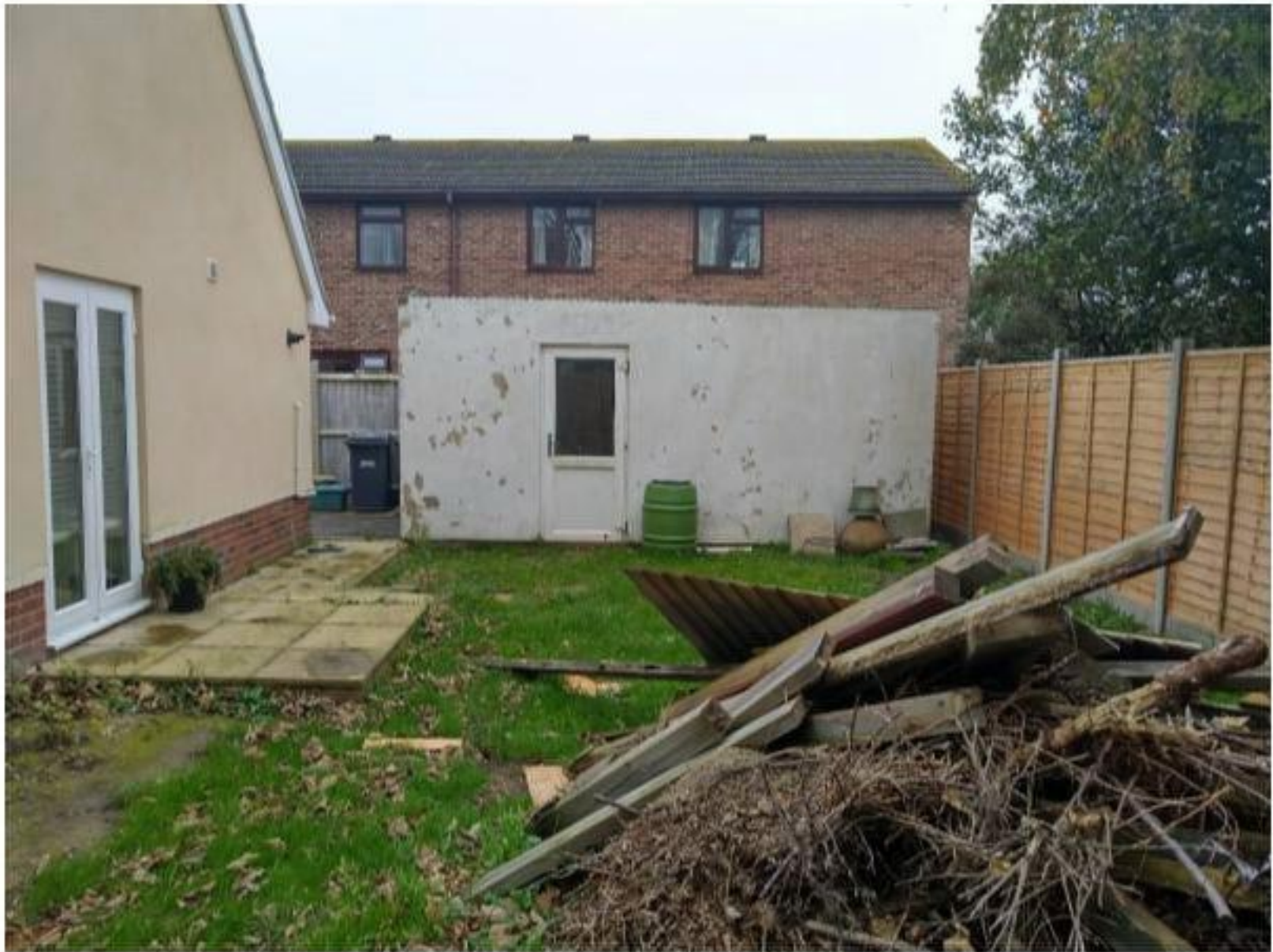
Photo 6: Side of Garage
