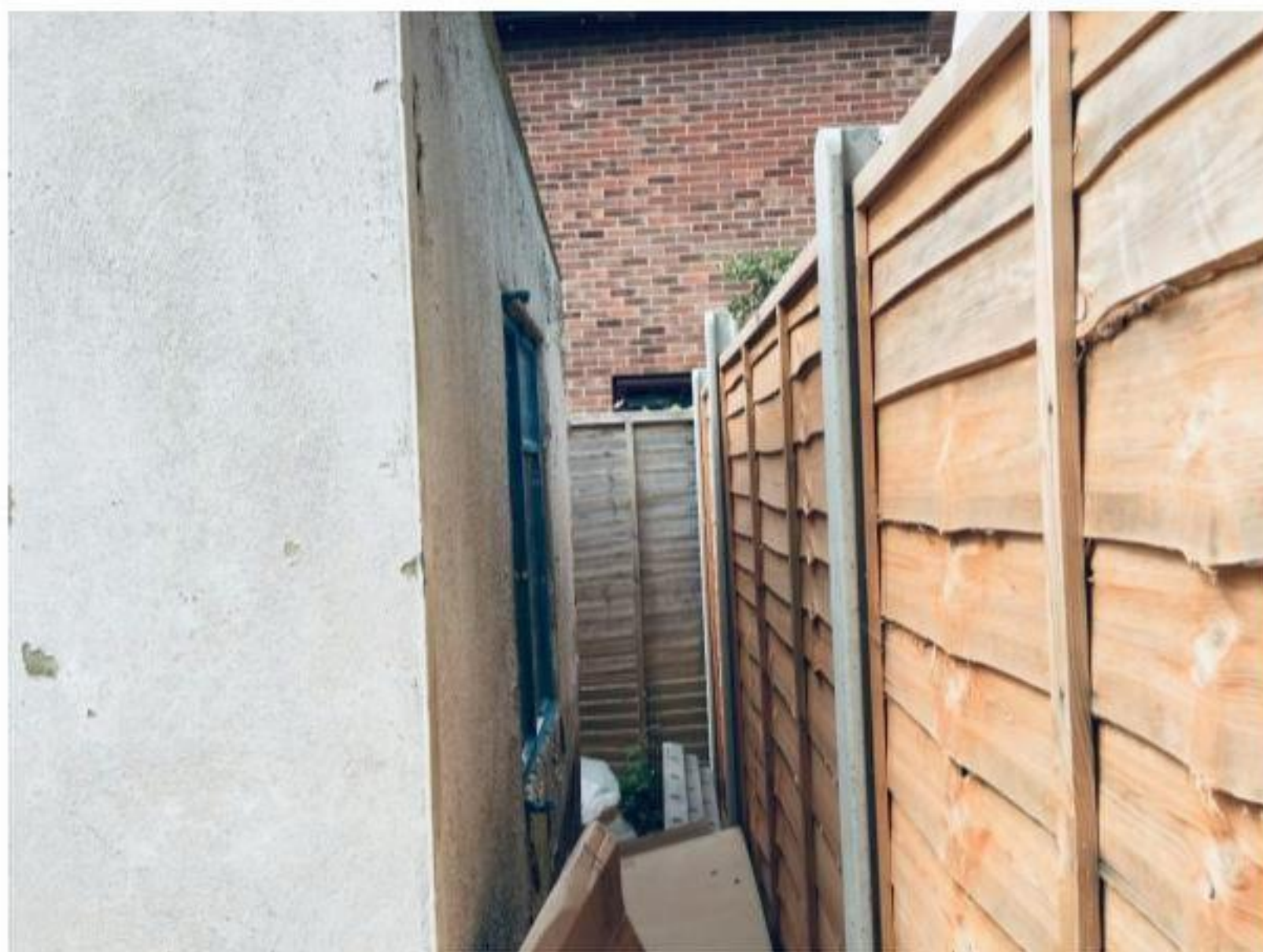
Photo 7: Shared boundary with garage
