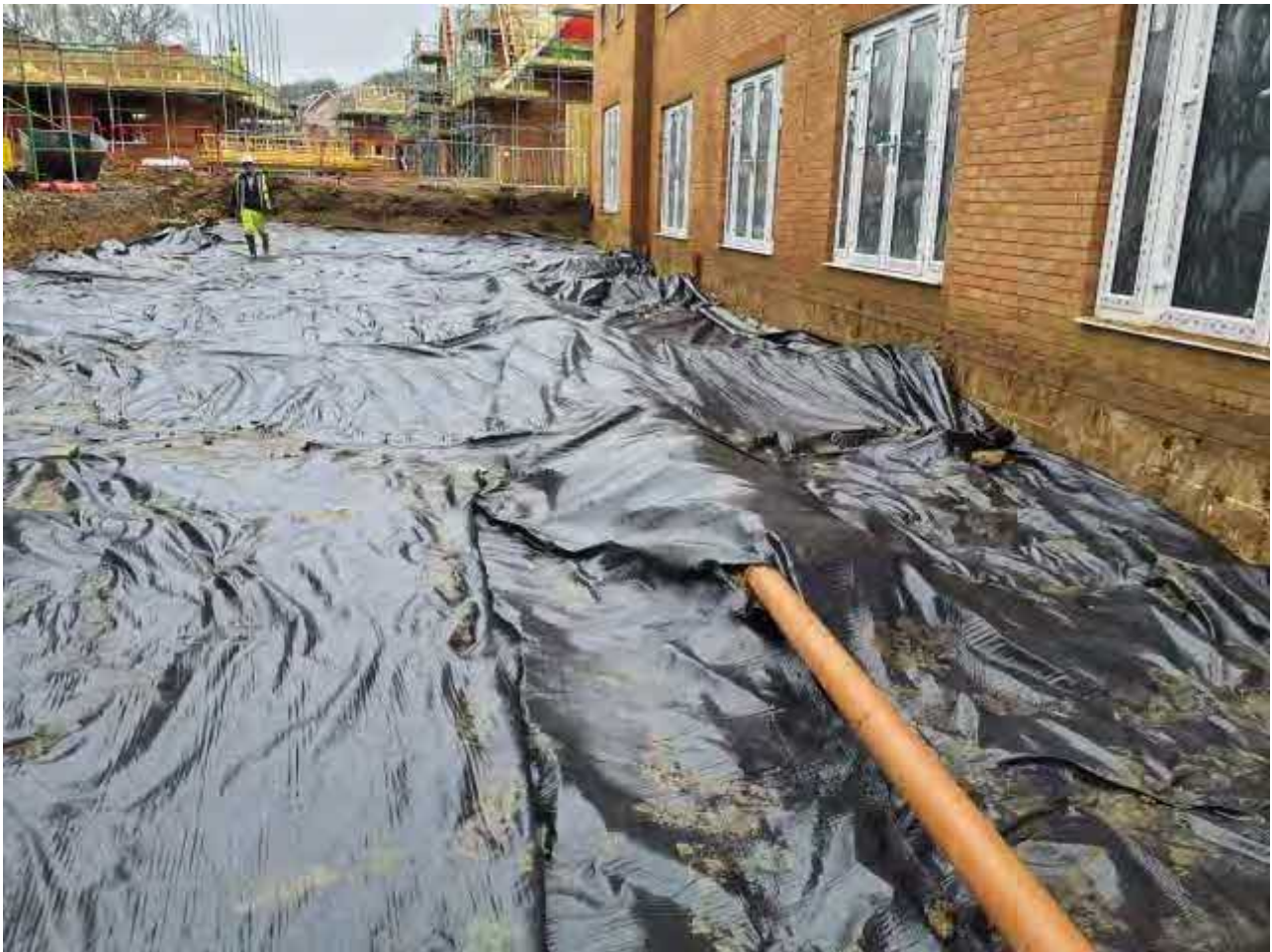
Plate 2 – View of reduced dig with black geotextile above in Plots 108-112
