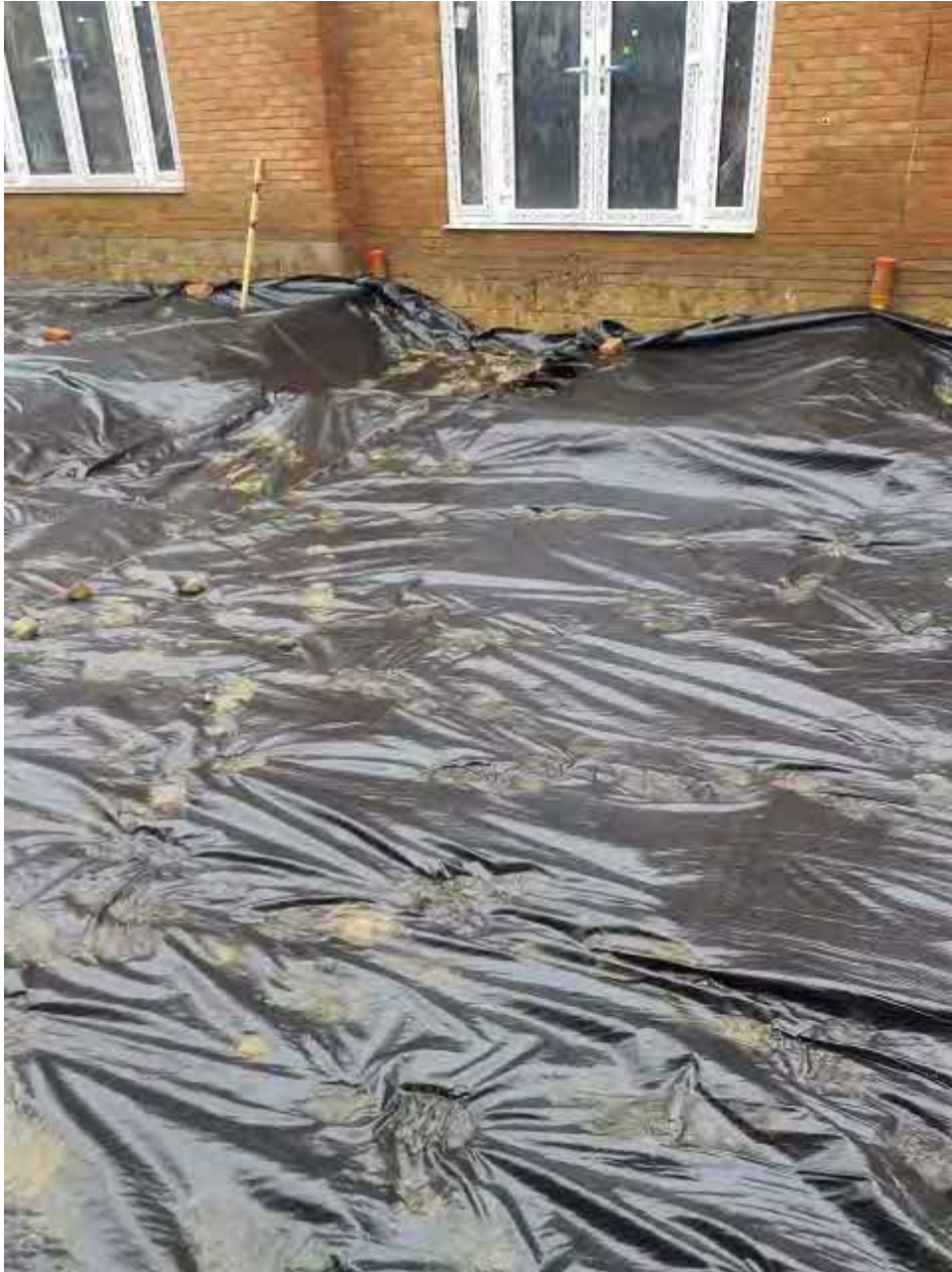
Plate 5 – View of reduced dig and black geotextile in Plot 111
