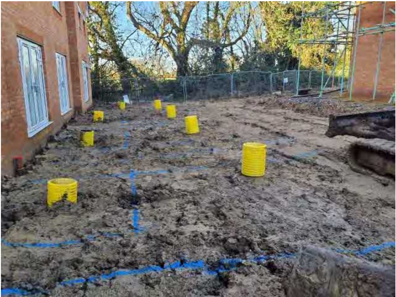
Plate 9 – View of subsoil installed across Plots 108-112
