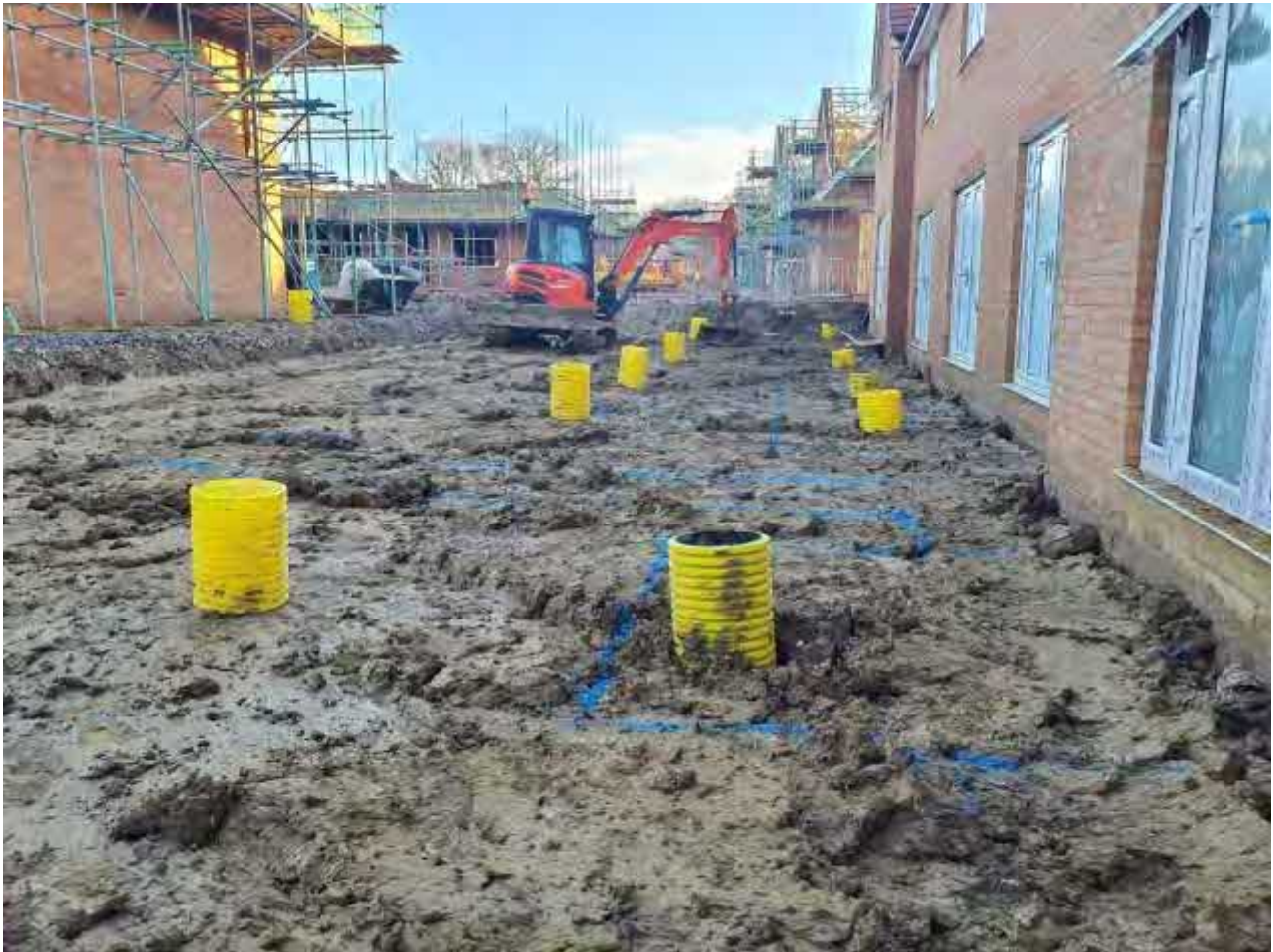
Plate 10 – View of subsoil installed across Plots 108-112
