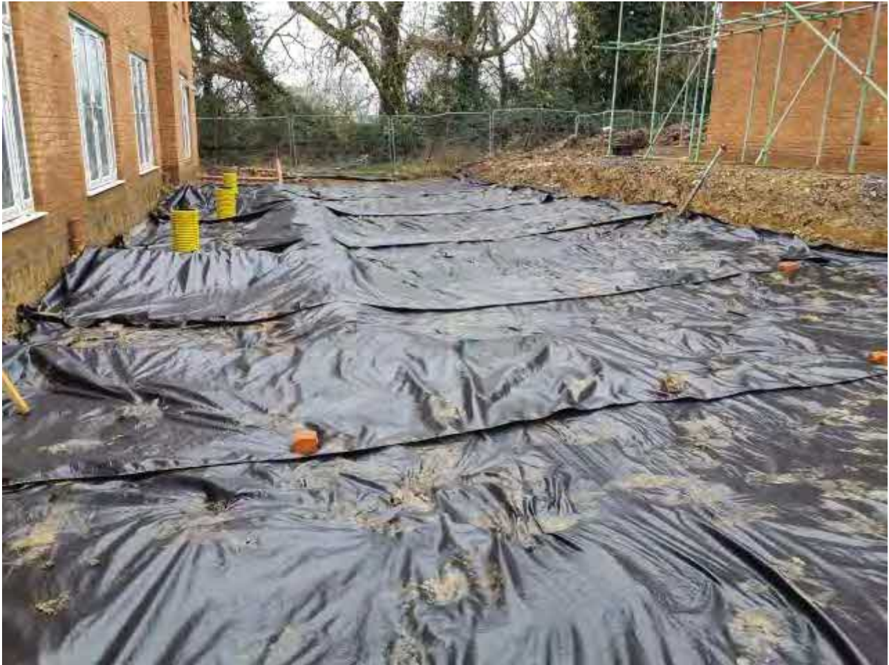
Plate 1 – View of reduced dig with black geotextile above in Plots 108-112
