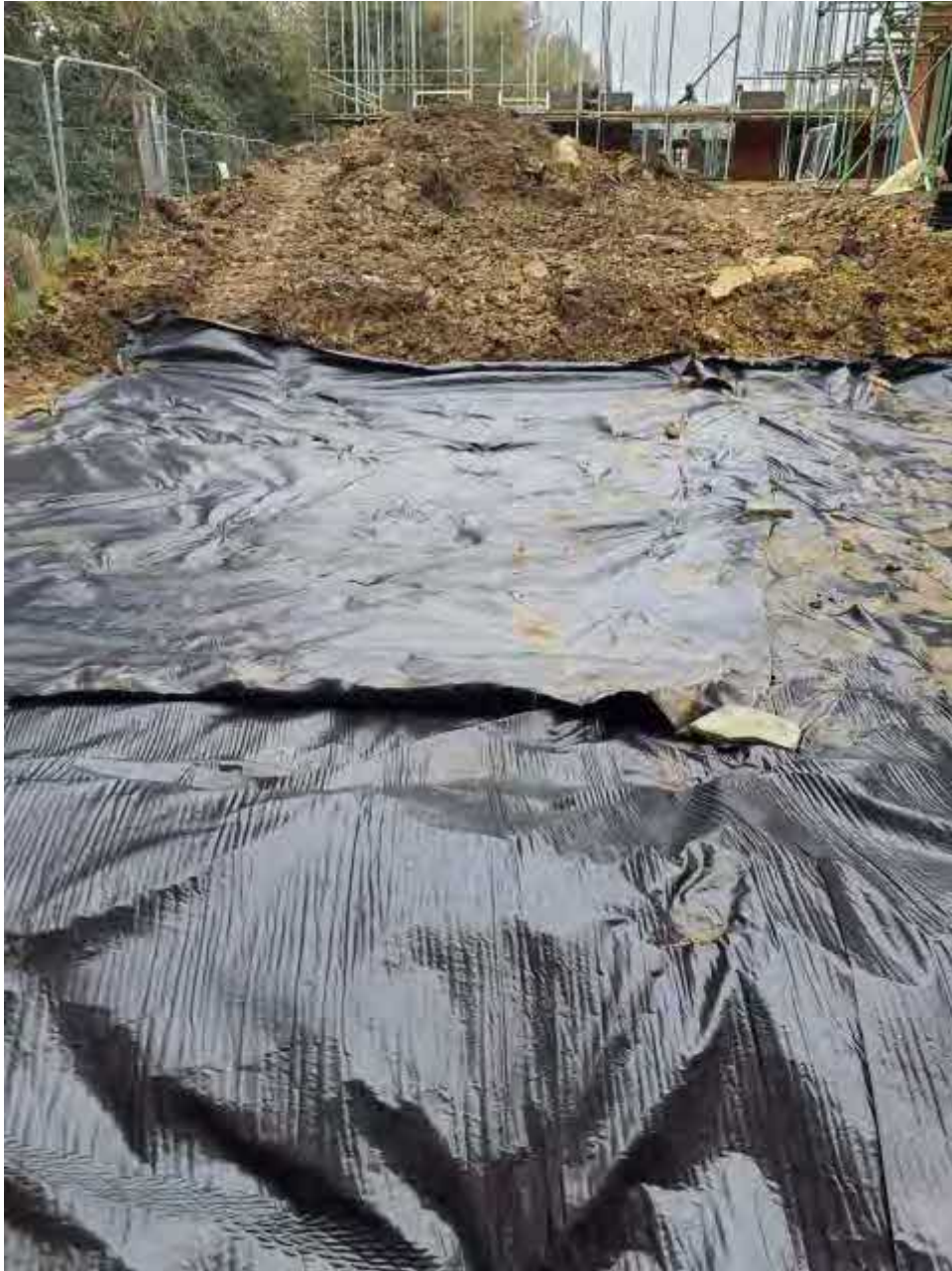
Plate 3 – Reduced dig and black geotextile in Plot 108
