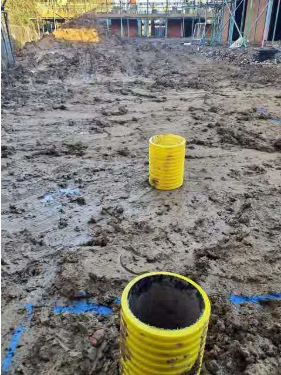
Plate 12 – View of subsoil installed in Plot 108
