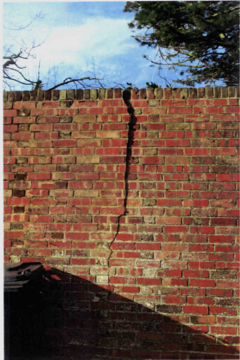
Photographs taken April 2021 - cracks have increased since then.
