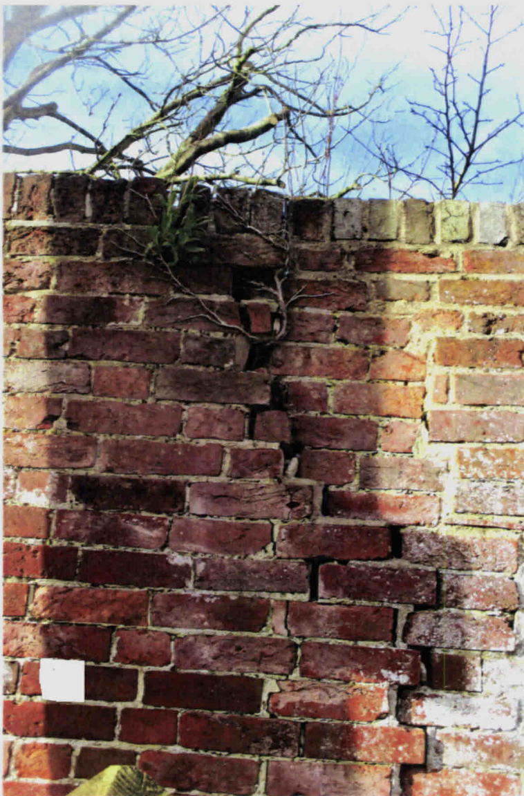
Photographs taken April 2021 - cracks have increased since then.
