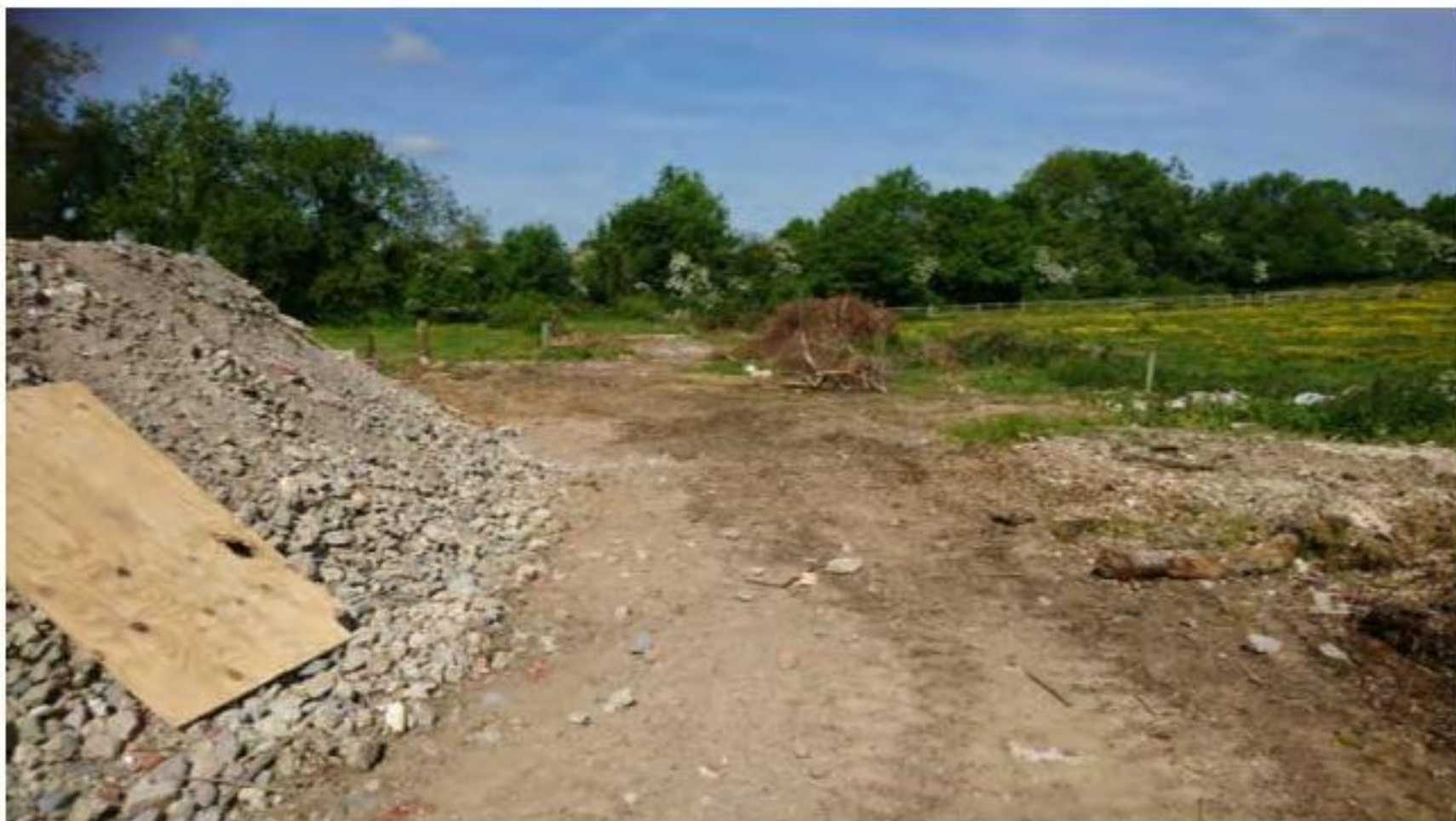
Plate 11 View west towards horse arena area
