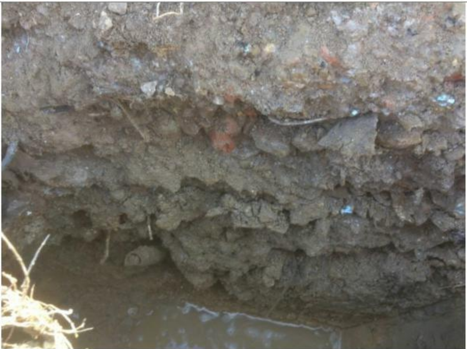
PLATE 4 – TP2 abandoned due to high, possibly due to water running along old pipe gravel surround
