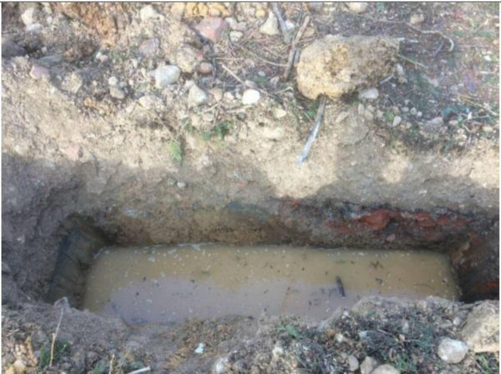
PLATE 3 – TP1 at start of soakaway test
